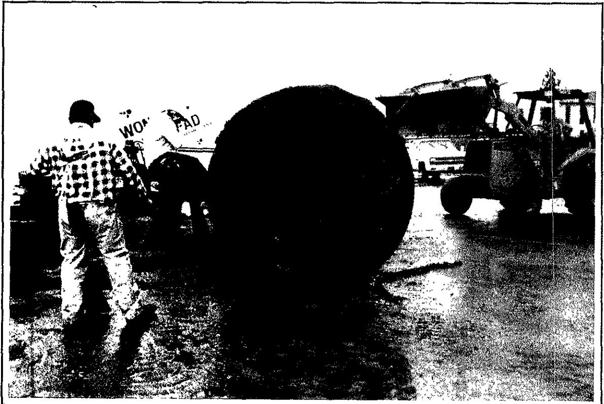
December 17, 1992: South end of UST immediately following removal
