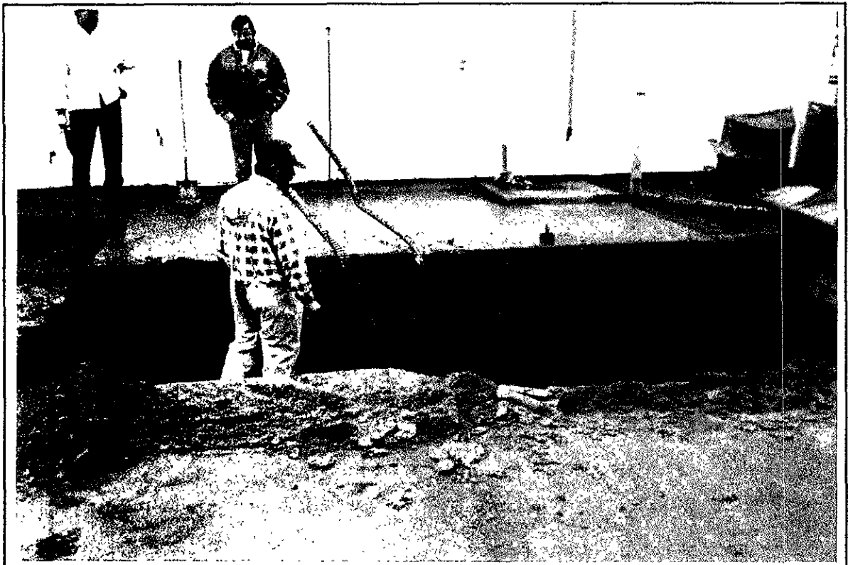
December 17, 1992: Product and vent lines during removal activities (facing west)
