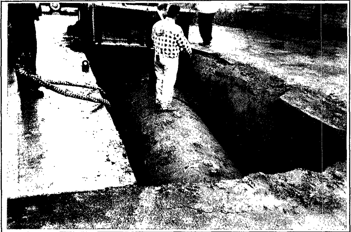
December 17, 1992: Top of UST during removal activities (facing north)
