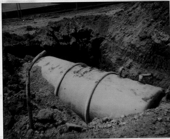
Chevron 19201 Center St, Castro Valley 1,000 gallon Waste Oil Tank
