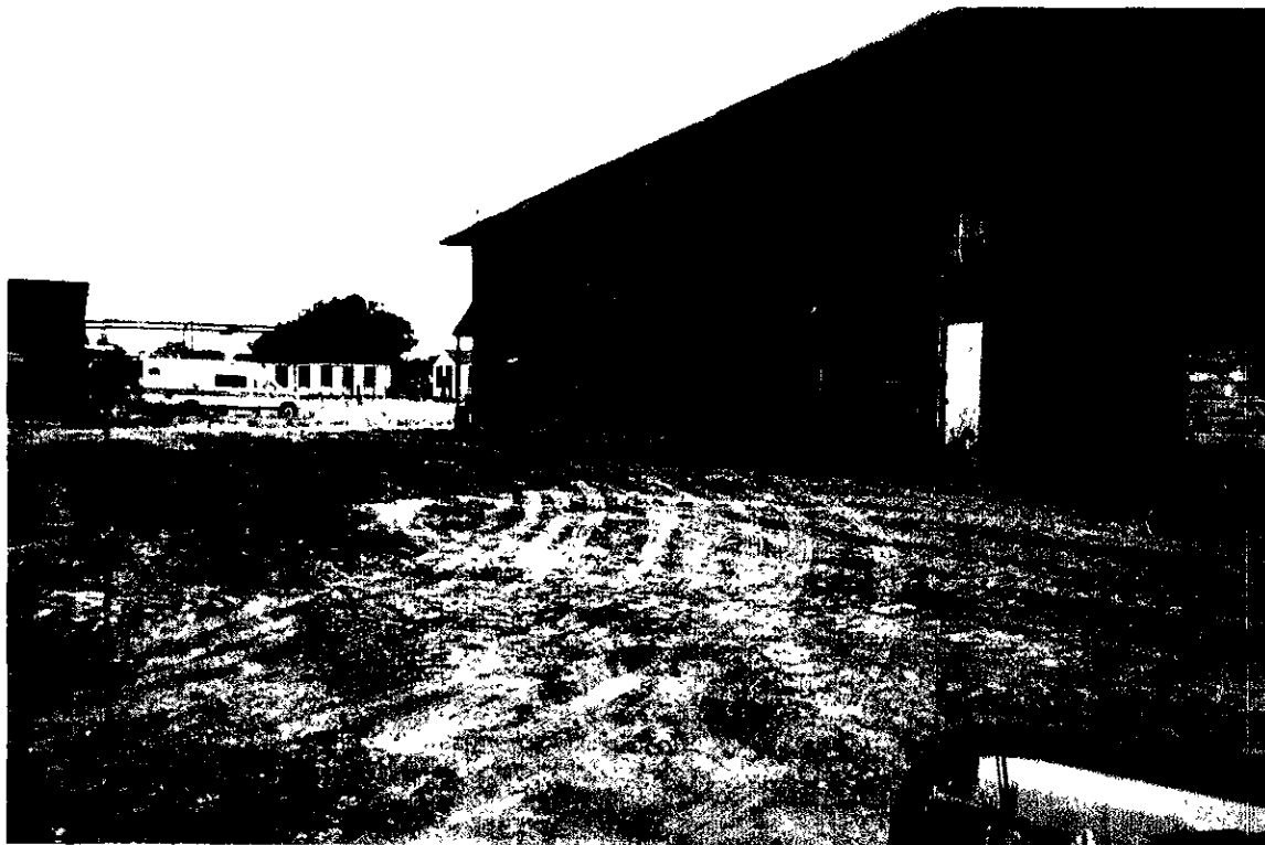
Plate 19 - Viewing toward northeast at final grade over the east portion of the former UST 18 & 19 excavation .
