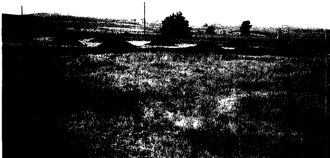
Plate 8 - Viewing toward east at spreading of stockpiled soil on the receiving field. Final approximate spread soil thickness was six inches.
