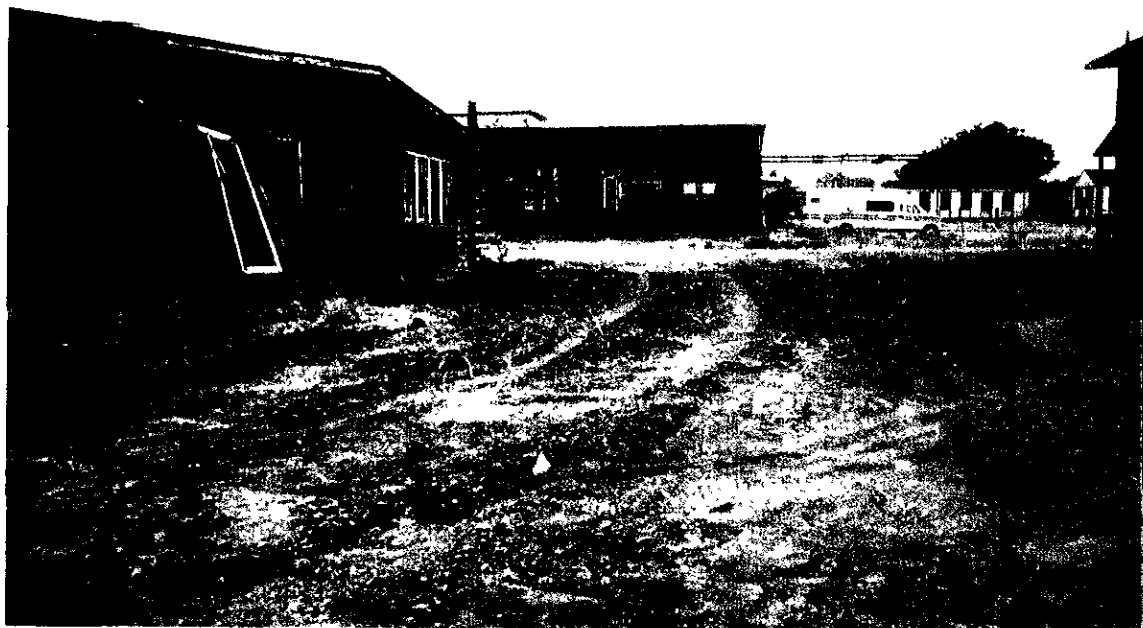
Plate 20 - Viewing toward north at final grade over the west portion of the UST 18 & 19 excavation.
