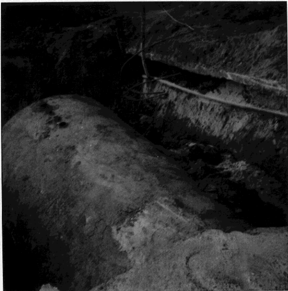
West side of Tank pit - gasoline 20009 Merland Av., Hayward 10-16-90
