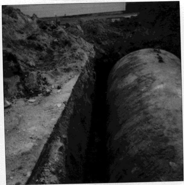
E. side of Tank Pit - Gasoline 20009 Merland Av., Hayward 10-16-90
