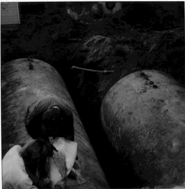
S. side of Tank pit - Gasoline 20009 Merland Av., Hayward 10-16-90
