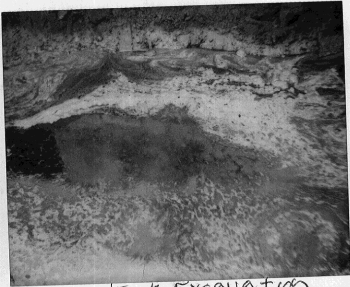
10000 GL Tank Excavation 2-7-91 10:30am Weyerhaeuser Co Alameda W. Faulhaber
