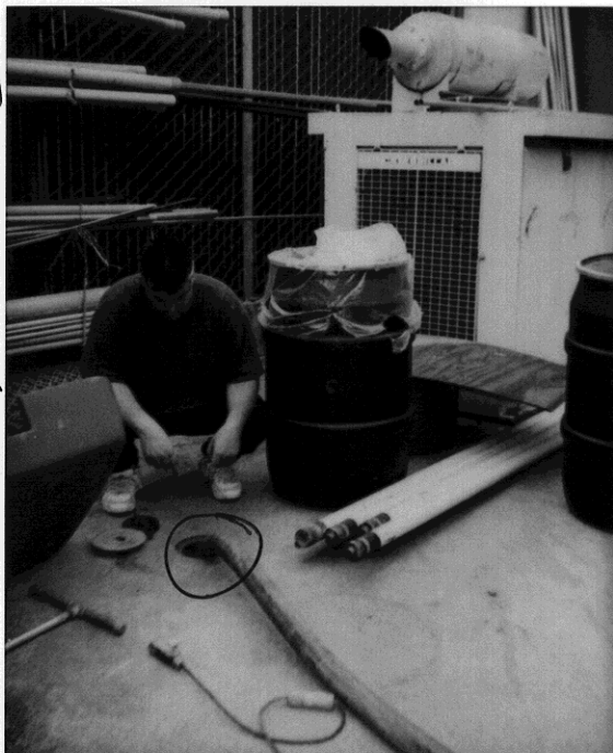
TANK BEING FLOED W/CEMENT
