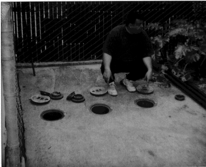
JUVENILE HAW TANK CLOSURE IN PLACE 6-22-98
