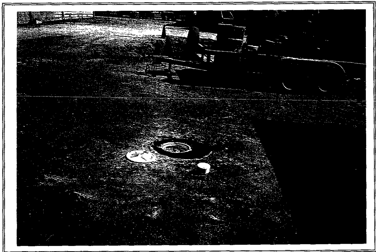
Photograph #9 Installation of PVC Casing for Dry Well
