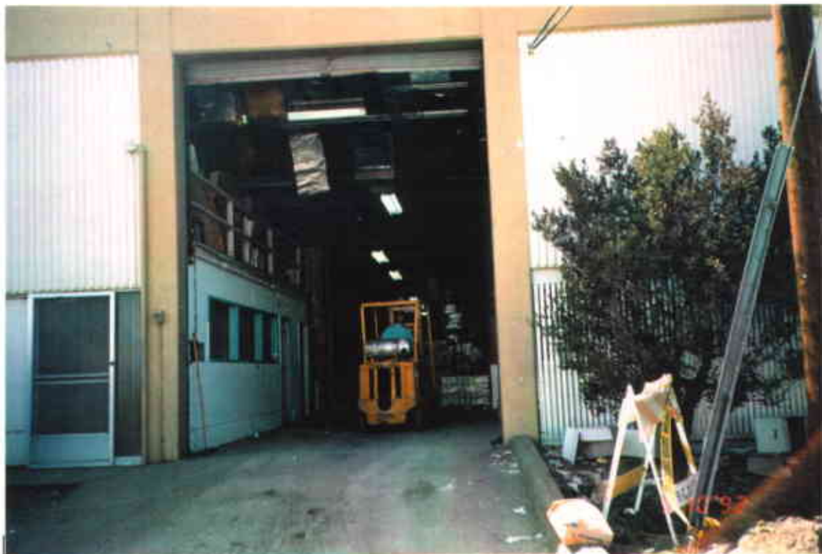
2. Front of Richards and Sterling (facing west), a ceramic and tile distributorship that leases a portion of the warehouse from Nady Systems, Inc.
