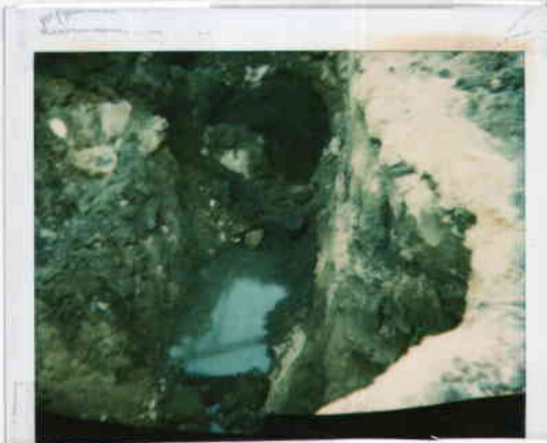
8/16/96 water in pit Omega Termite 11518201208-24 2028 7046 COPIES & ENLARGEMENTS CALL 800-421-1030 807-75th Ave
