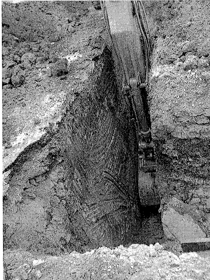
Photograph 2: Pre Trenching activities prior to setting shoring.
