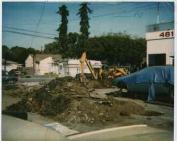
Former tank pit
