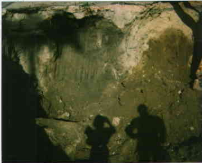
508 E Lawelling, S.L. 4/14/99 South Sidewall. No longer staining where it used to be during 09318221467-2 tank removal in Aug '98 0547 1730 Juliet Shinn
