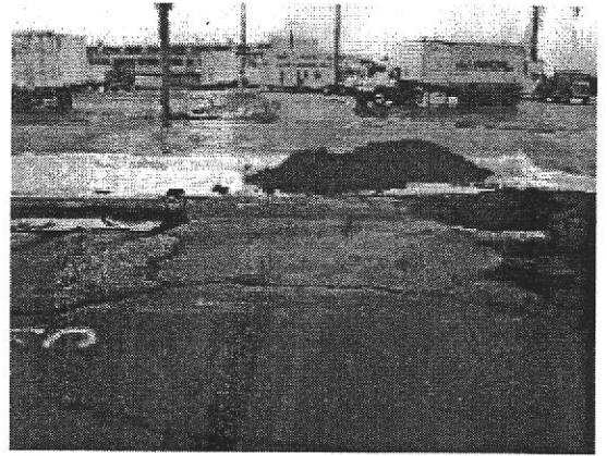
#2 Soil stockpile located adjacent to GAIA TP-5
