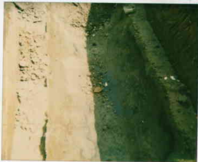
Pit of 10,000-gal gas UST. Lim/Former Exxon, 250-8th St., Oak 94607 5-7-92 JEberle
