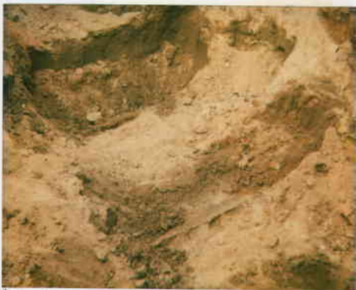
Pit from 3 500-gal gas tanks. Lim/Former Exxon, 250-8th St, Oak 607 5-7-92 JEberle
