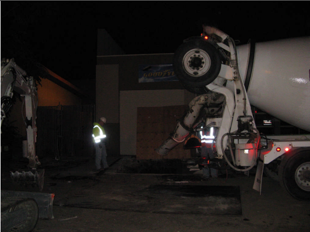
View of backfilling of excavation.
