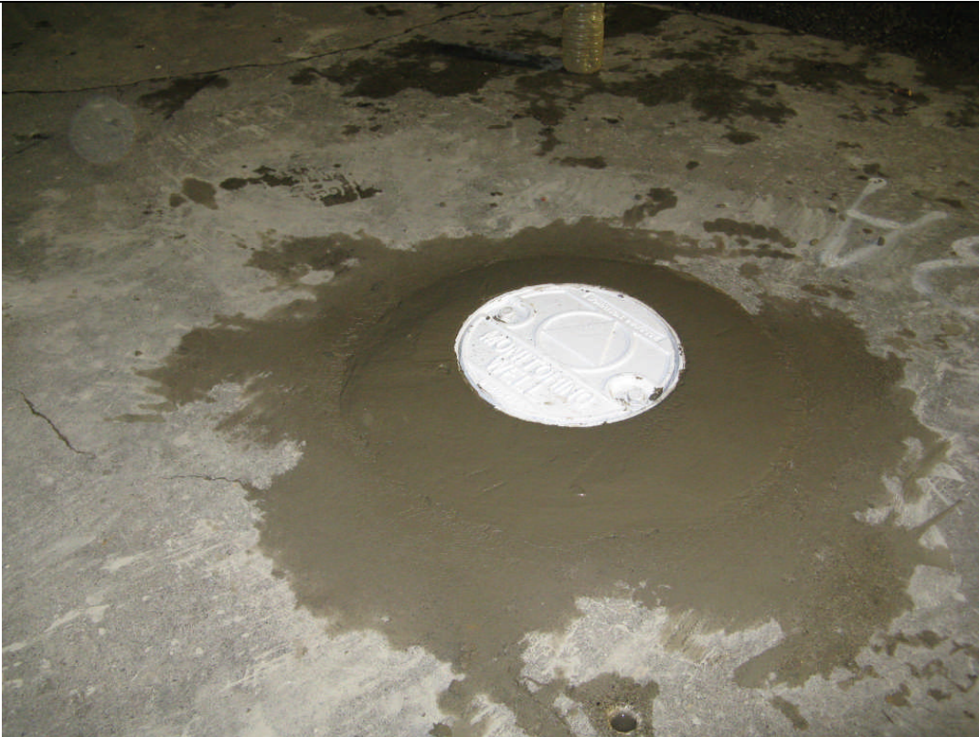
View of completed groundwater monitoring well MW-5.
