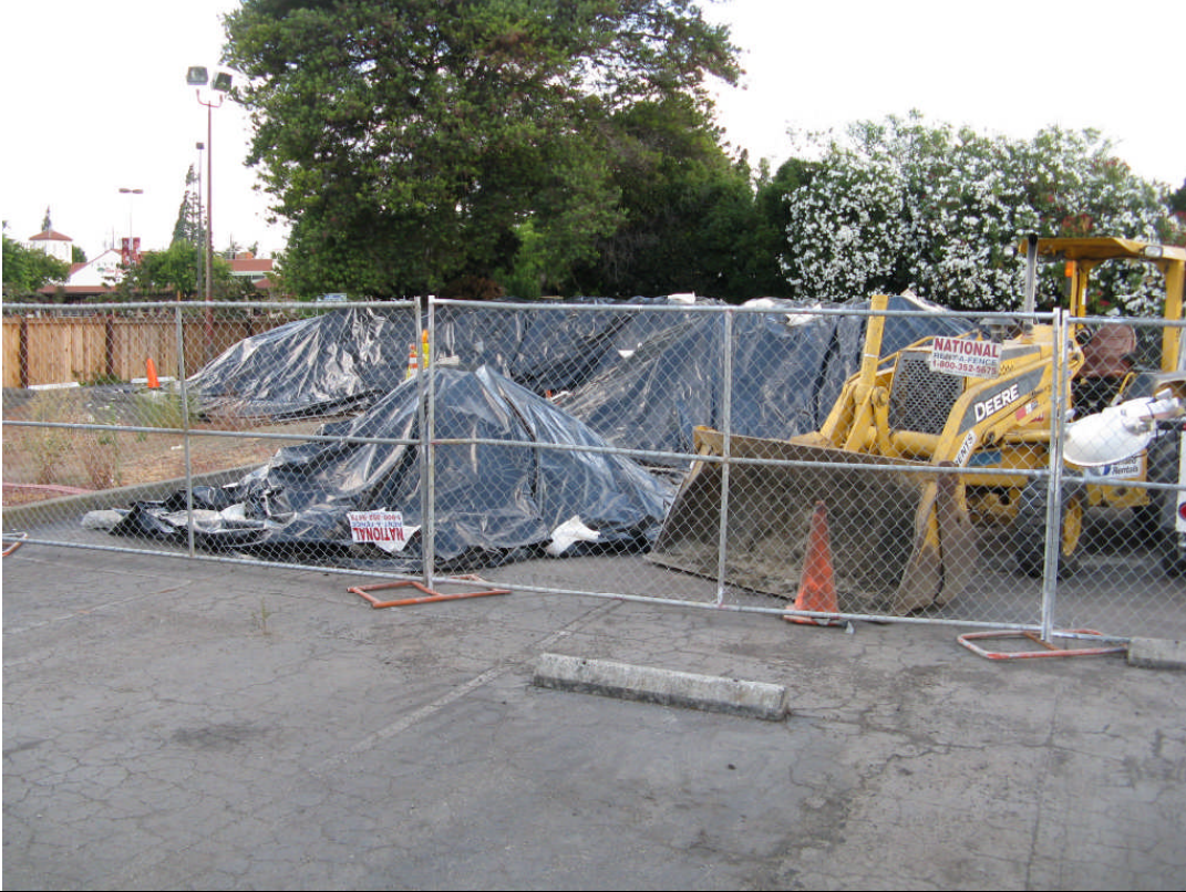
View of the soil stockpile and equipment.
