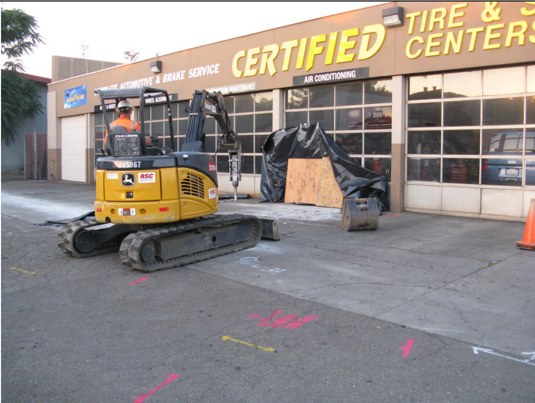
View of jack hammering of concrete prior to excavation.
