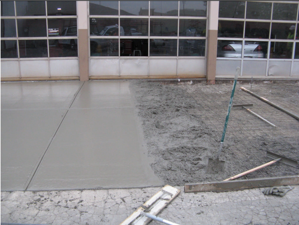
View of the concrete restoration activities.
