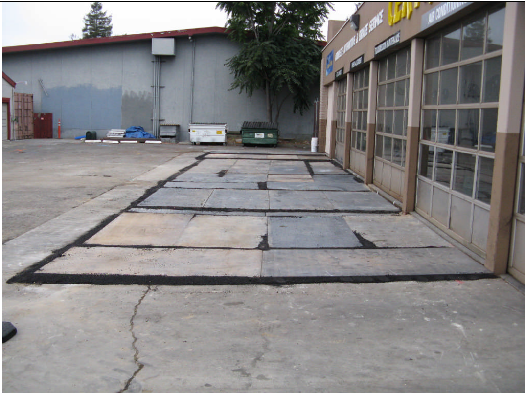
View of secured excavation during business hours.
