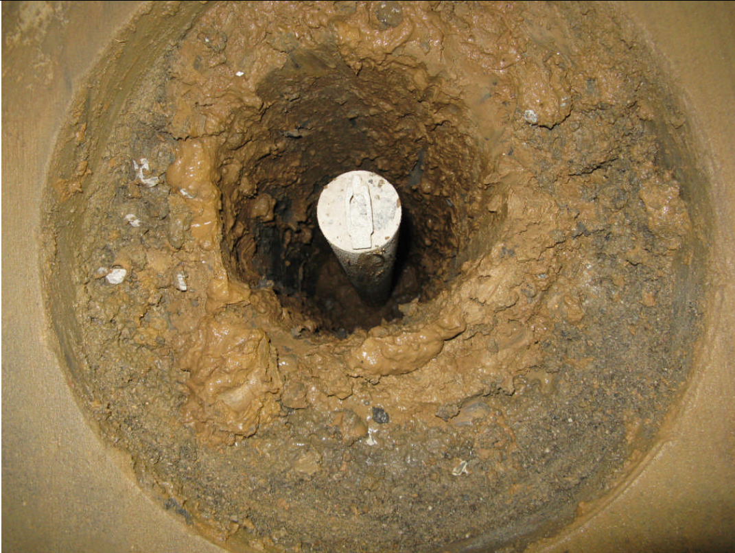
View of the well casing for groundwater monitoring well MW-5.
