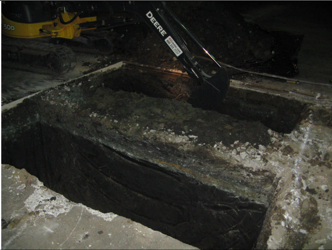
View of the excavation activities.
