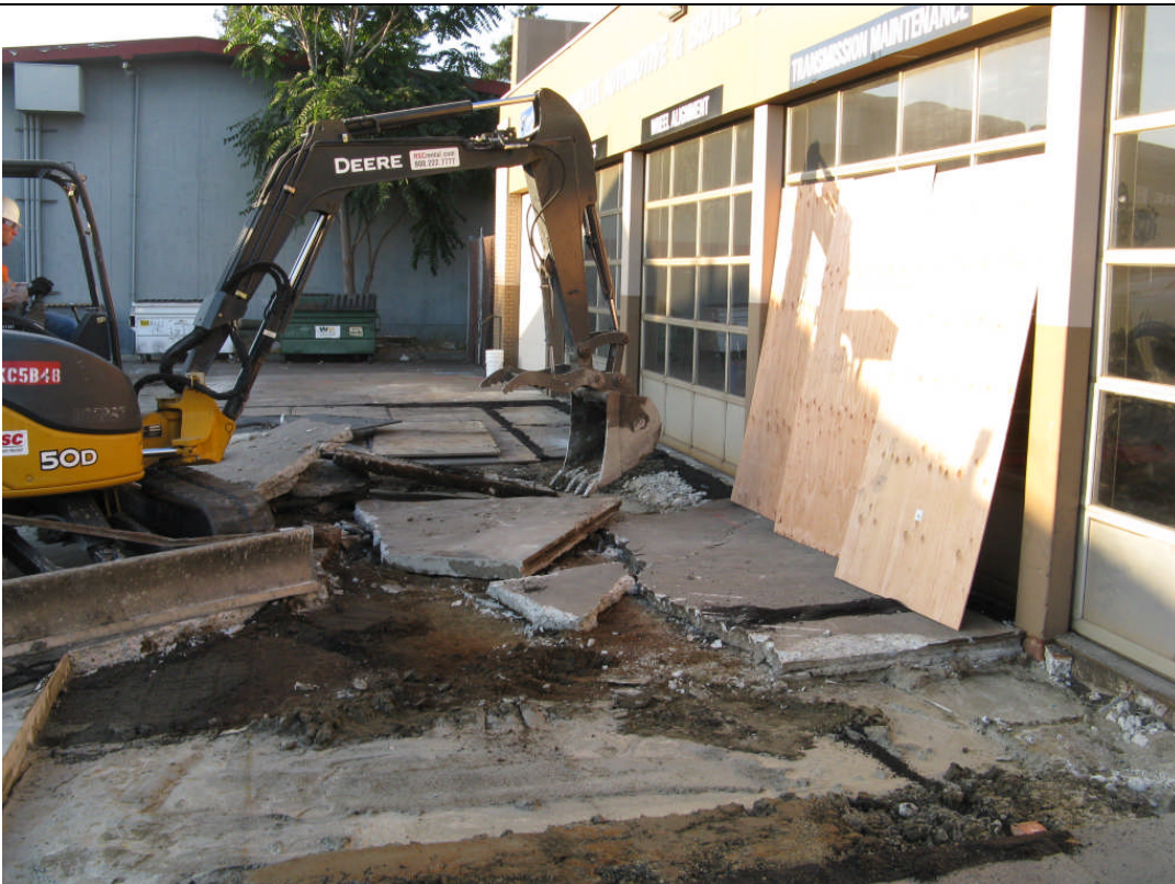
View of removal of concrete prior to excavation.
