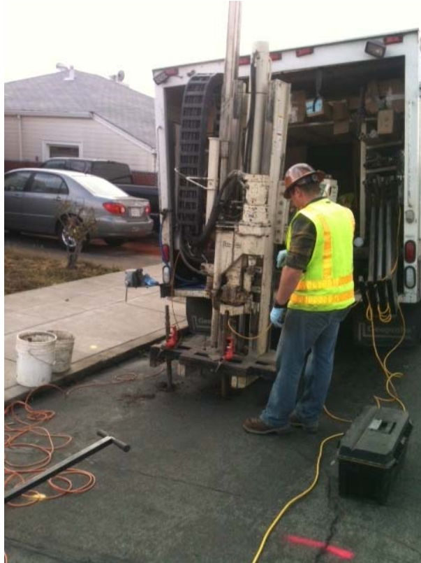
Plate 3. Fisch Drilling on CPT/MIP-10
