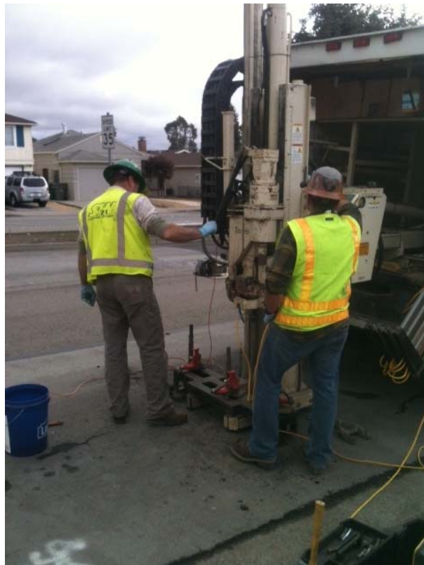
Plate 2. Fisch Drilling driving down for CPT/MIP-15
