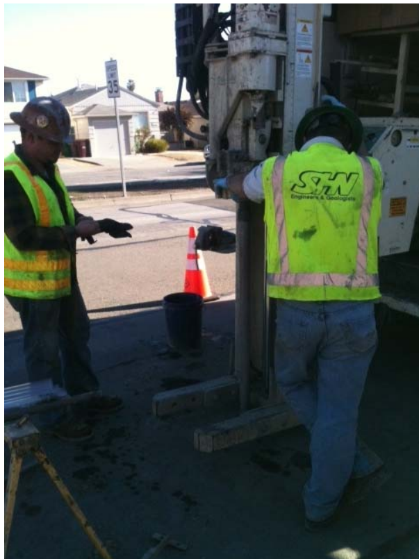
Plate 6. Fisch Drilling drilling on CPT-MIP-17
