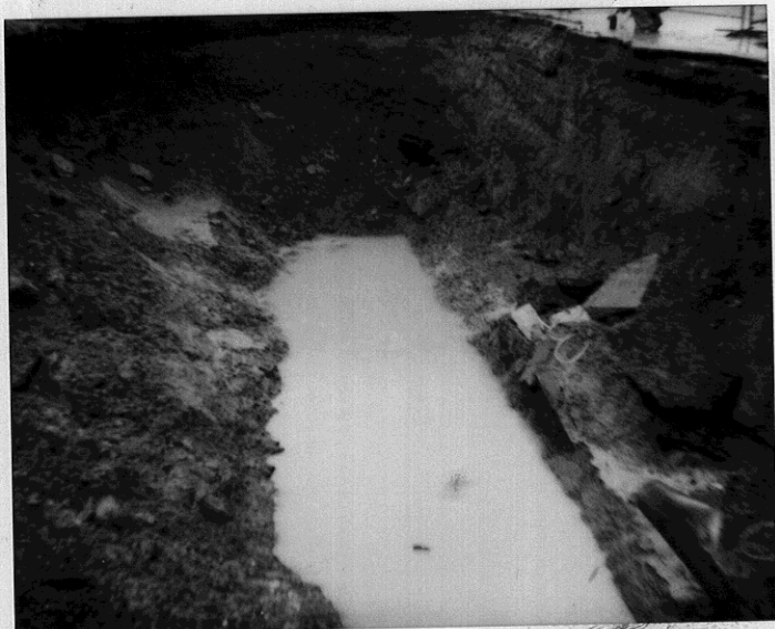
Open pit where 20K Gal was was removed. 2/23/93. Geo. H. D. Jeff S. CAMP PARKS
