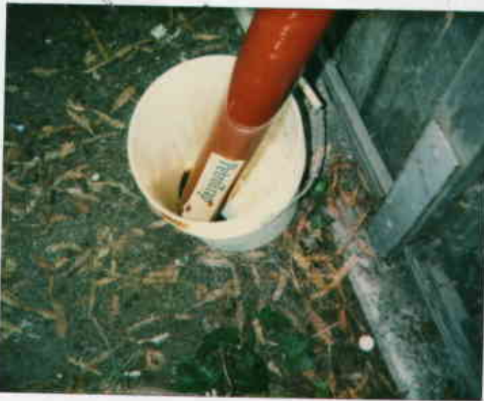
Shell 6039 College Ave Oakland
