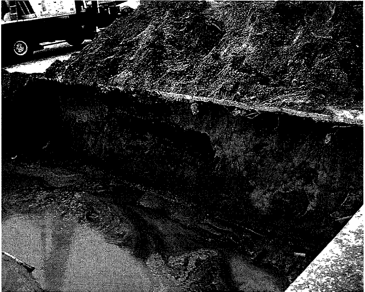
Figure 2 - Waterline of tank excavation shows the change of soil types in the sidewall excavation. Also a froth on the water surface is indicative of organic material breakdown.
