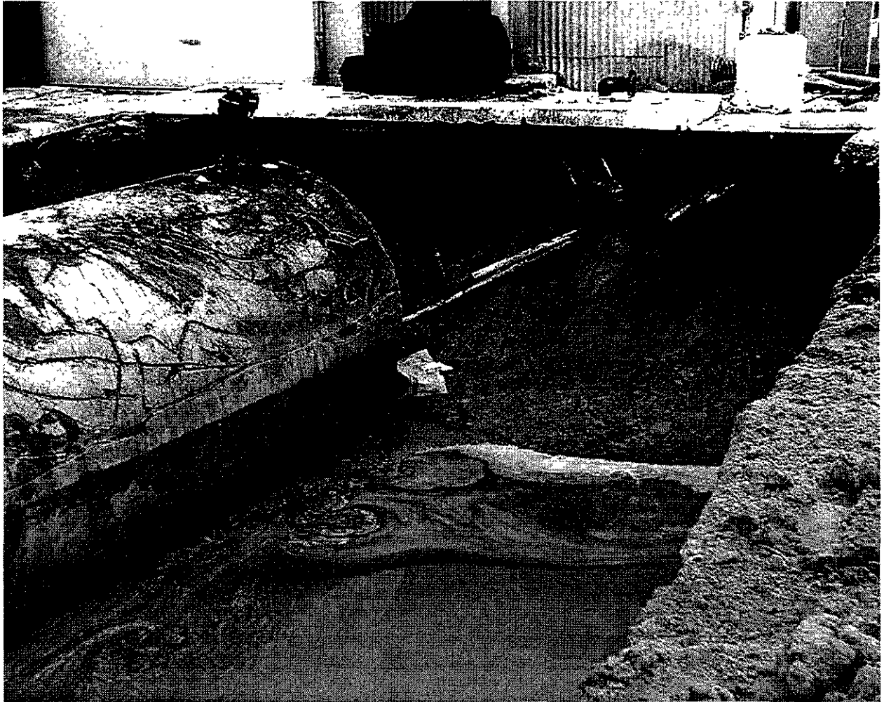
Figure 3 - The tanks were in very good condition. The water line on the tank indicates that the water level fluctuated; probably due to tidal action.
