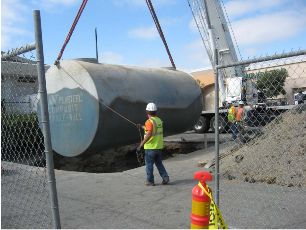
Removal of diesel UST
