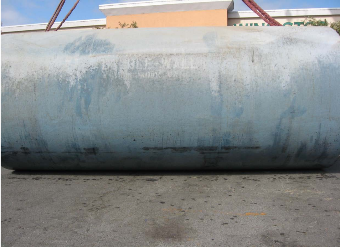
Removal of diesel UST
