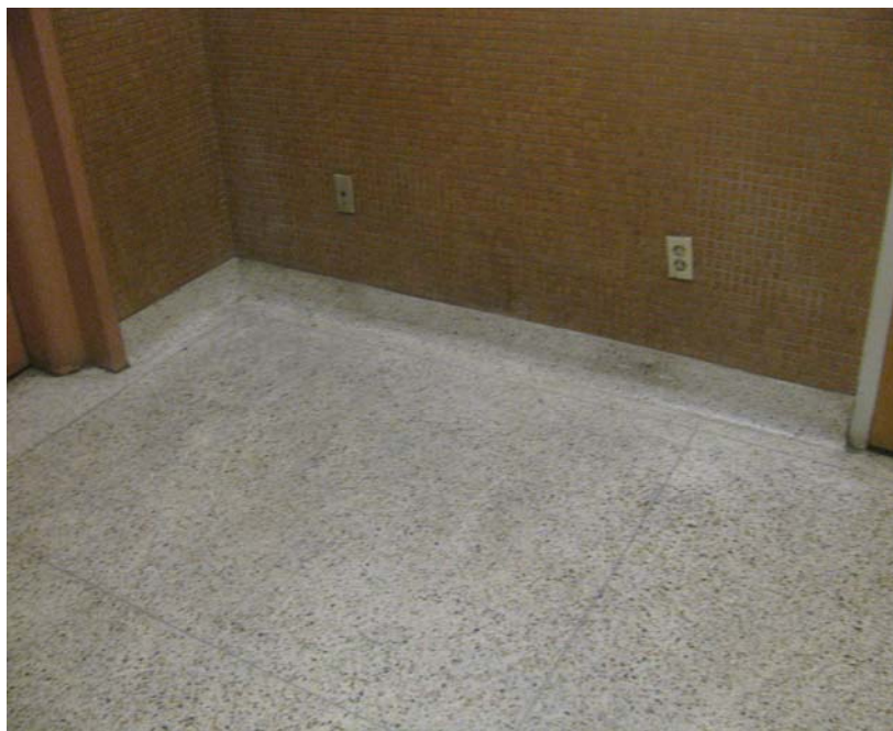
Plate 4. Wall between elevator and nearby door
