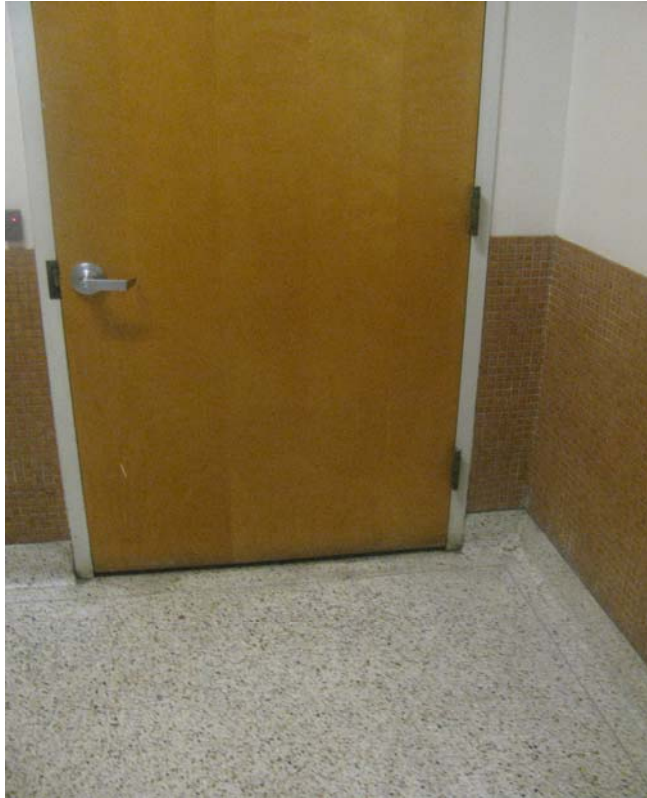
Plate 3. Door near elevator cars
