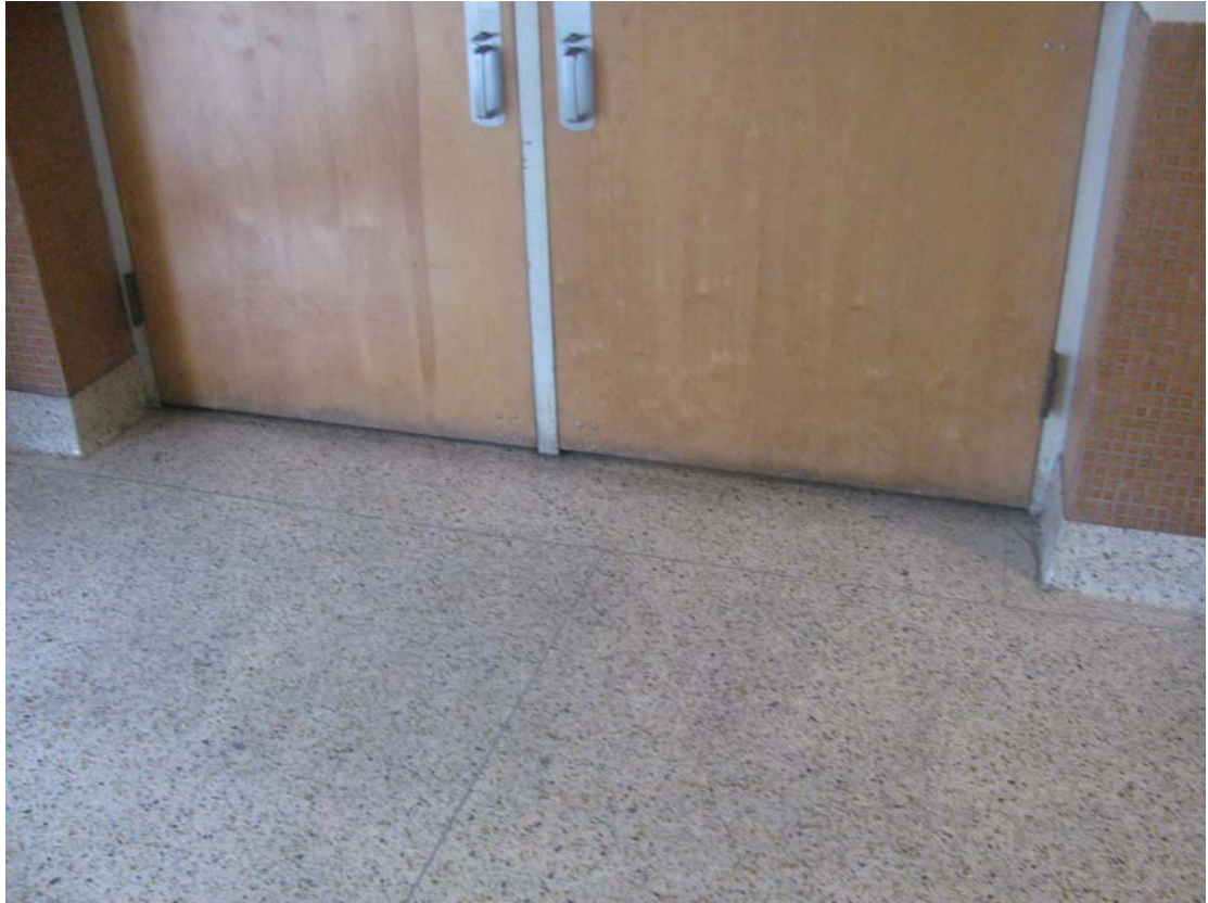
Plate 5. Door way between elevator cars and front entrance of building
