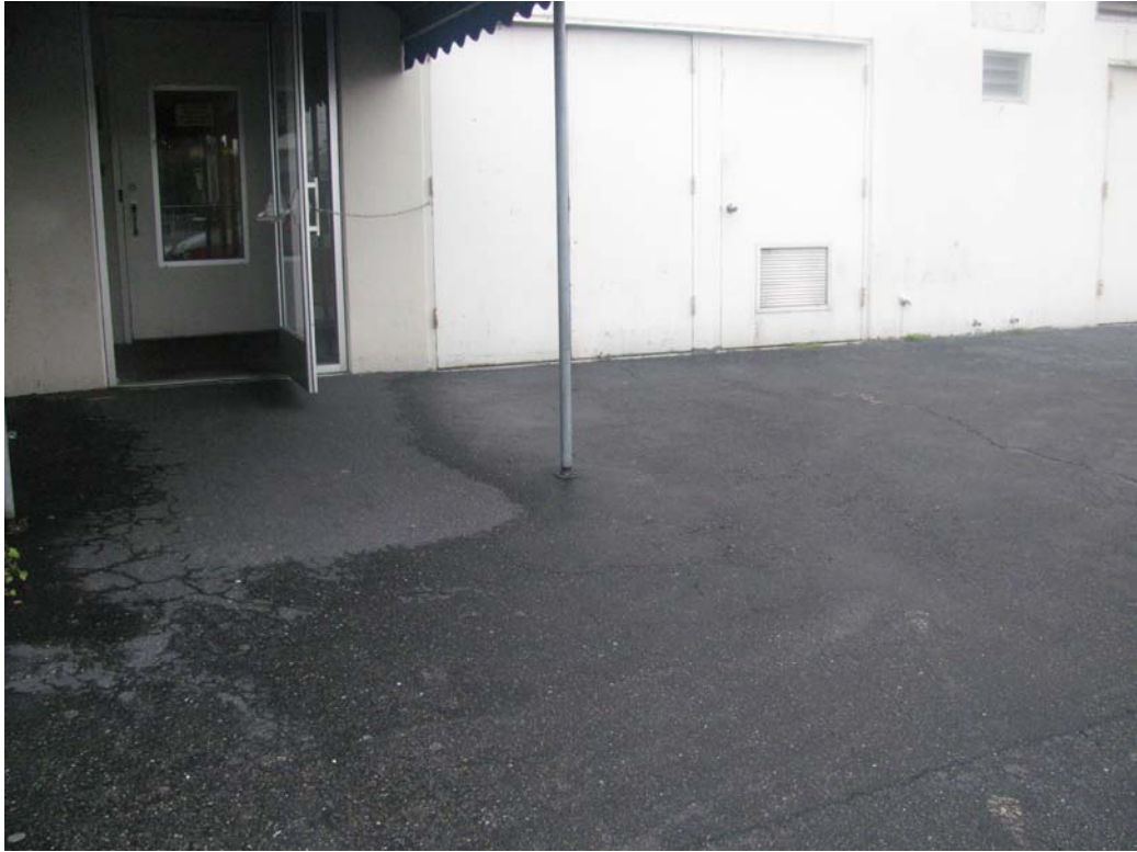
Plate 11. Rear entrance to Red Cross building, parking lot, Manila side
