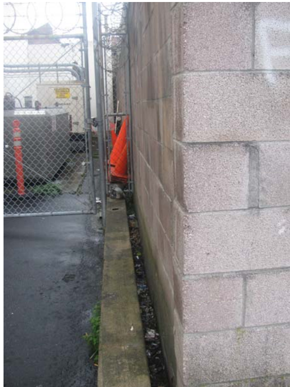
Plate 19. Alleyway between Red Cross and 3820 Manila Avenue (view south/southwest)
