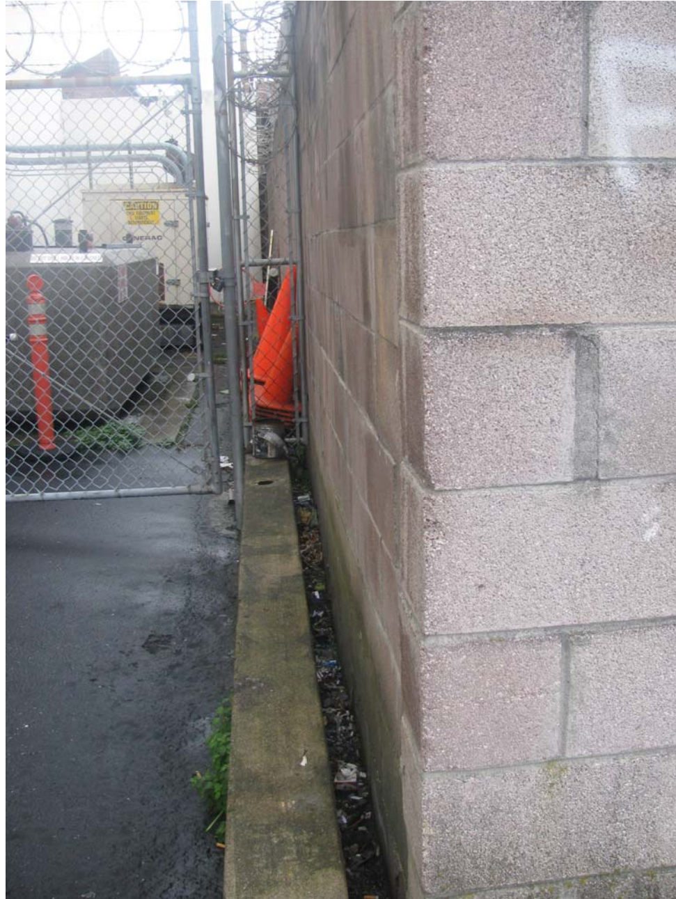
Plate 15. Retaining wall and wall, boundary with Glovatorium and Red Cross building
