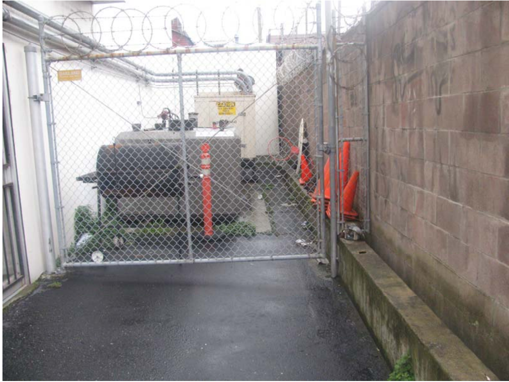
Plate 18. Alleyway between Red Cross and 3820 Manila Avenue (view south/southwest)
