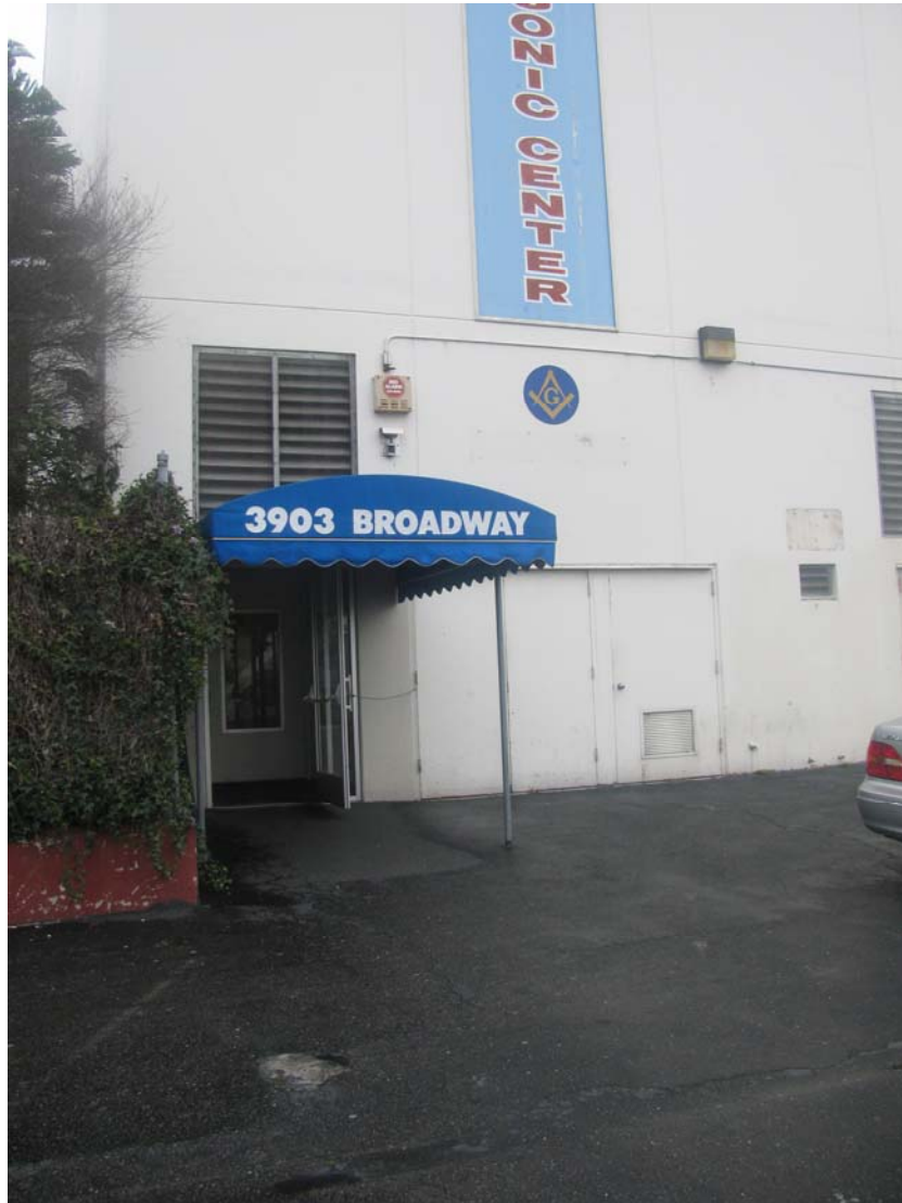
Plate 17. Rear of building
