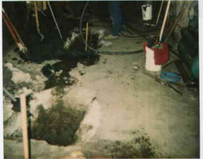
Glovatorium 305 Broadway 6/9/97 Top of USB in "man" walkway uncovered to facilitate pressure cleaning and video cam inspections of their interiors.
