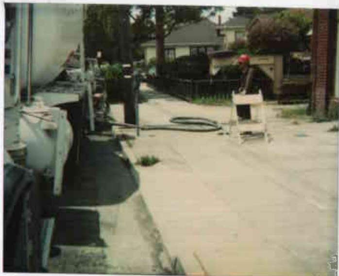
Filling 38 th street USTs. Glenview 6/11/97
