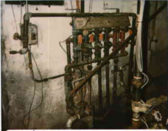
Glovatorium 3815 Broadway Oakland
