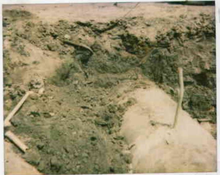
Tank C (SUL) strong tankage in the piping 5/18/94
