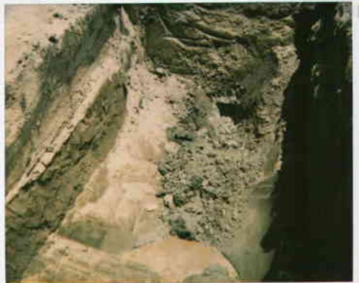
5/20/94 ST10567 DIESEL TANK EXCAVATION
