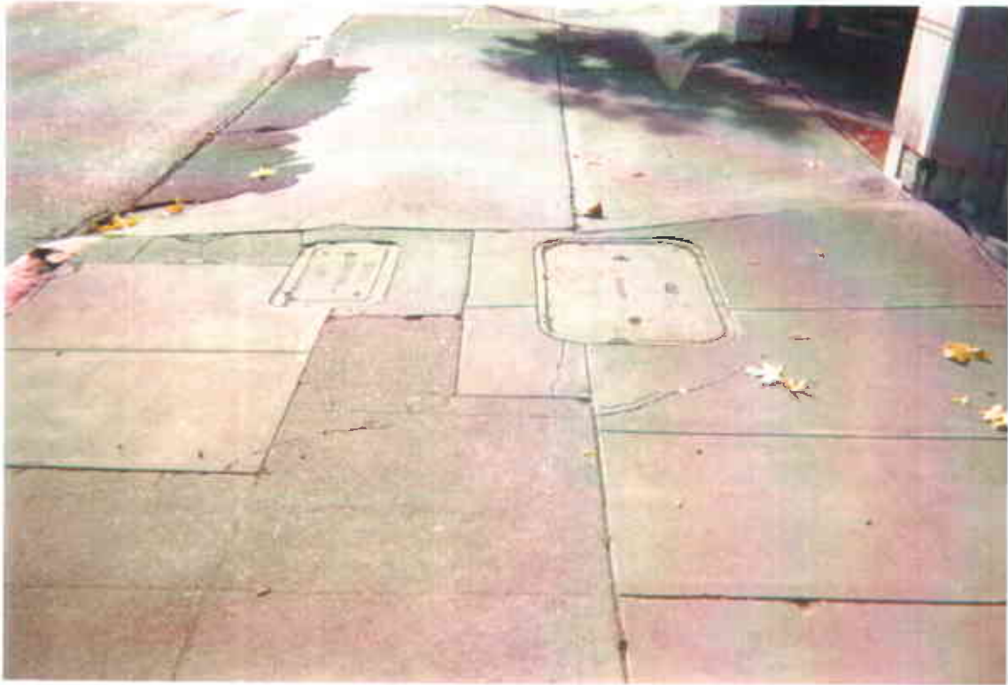
13. Electrical and street light utility boxes located at southwest corner of site
