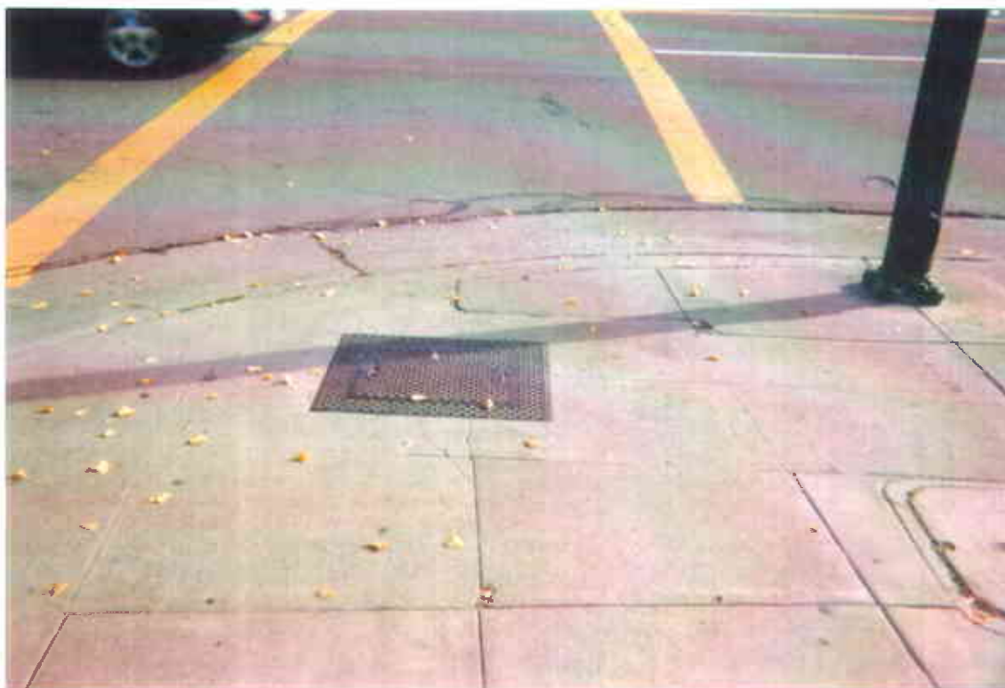
11. Unknown utility vault box located at southeast corner of site.
