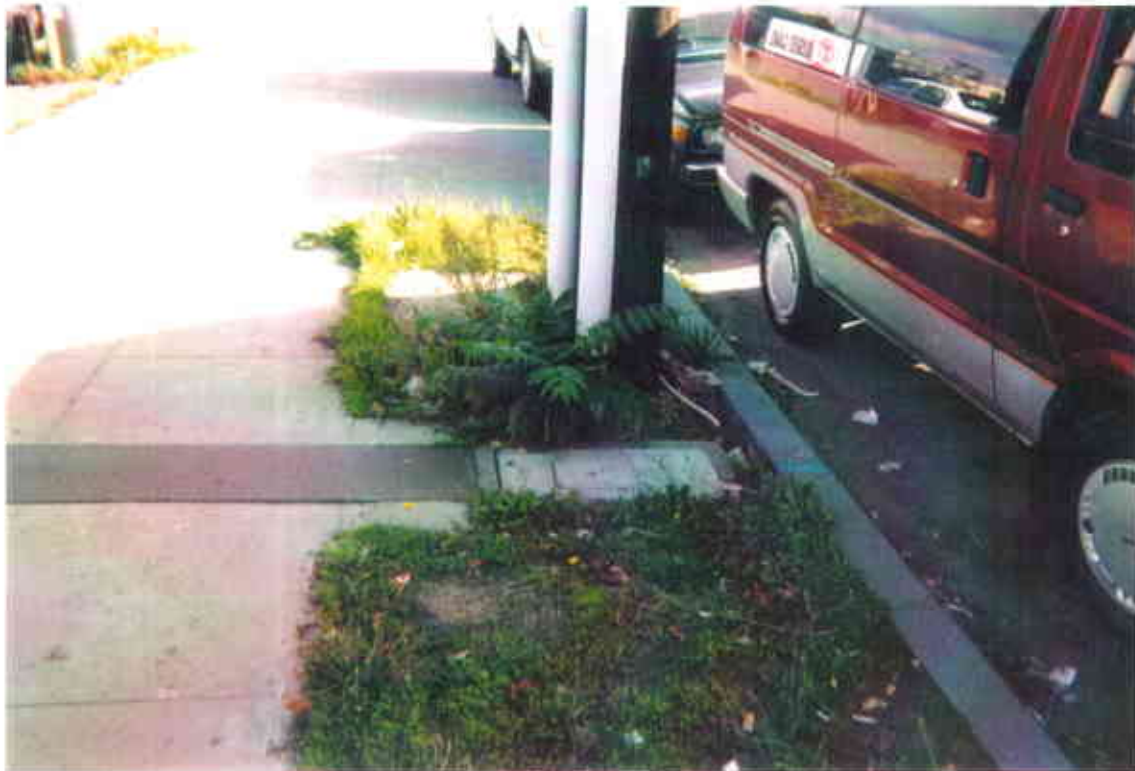
19. Water meter vault box located along south property boundary of 1601 Park Street (Former Chevron No. 9-4463).
