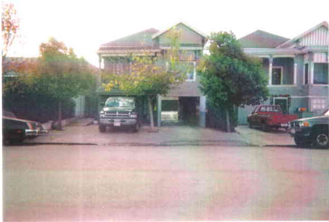
7. Residence with basement located at 2329 Eagle Avenue, approximately 20 feet north of site
