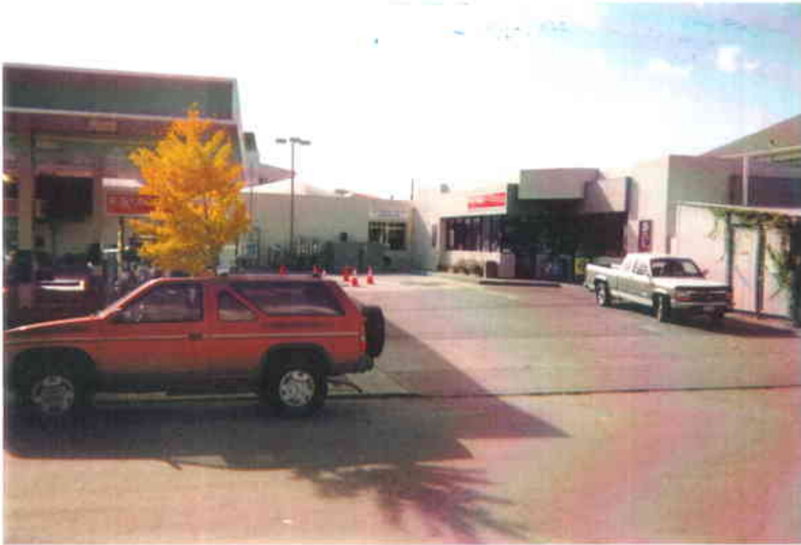
5. Front half of station building facing west
