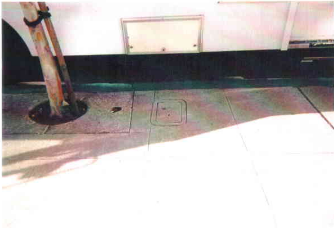
15. Water meter vault box located in sidewalk in front of 1719 Park Street, approximately 35 feet southwest of site.
