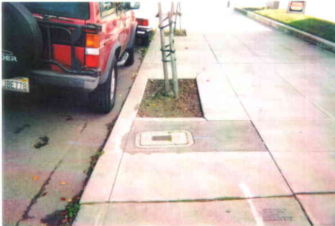
10. Water meter vault box along east property boundary
