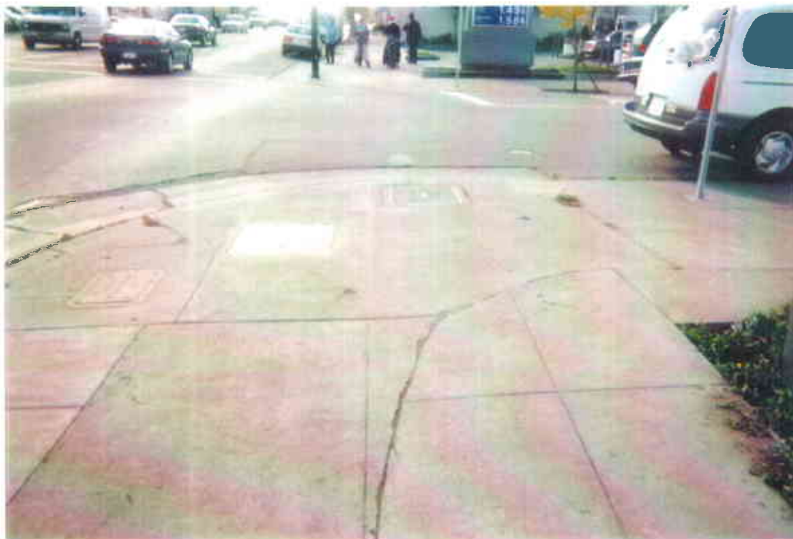
18. Two electrical and one unknown utility vault box located near the southeast corner of the property located at 1601 Park Street (Former Chevron No. 9-4463).
