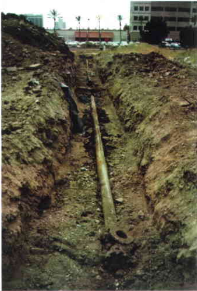
Photograph #4 Exposed 6-inch product pipe (looking west).
