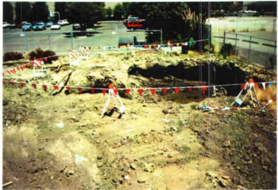
Photograph #5 Southeast excavation (looking east)
