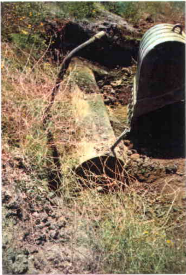
Photograph #1 Exposed central UST (looking south)
