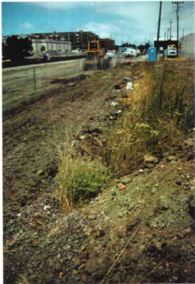
Photograph #6 View of former railroad siding (looking north).
