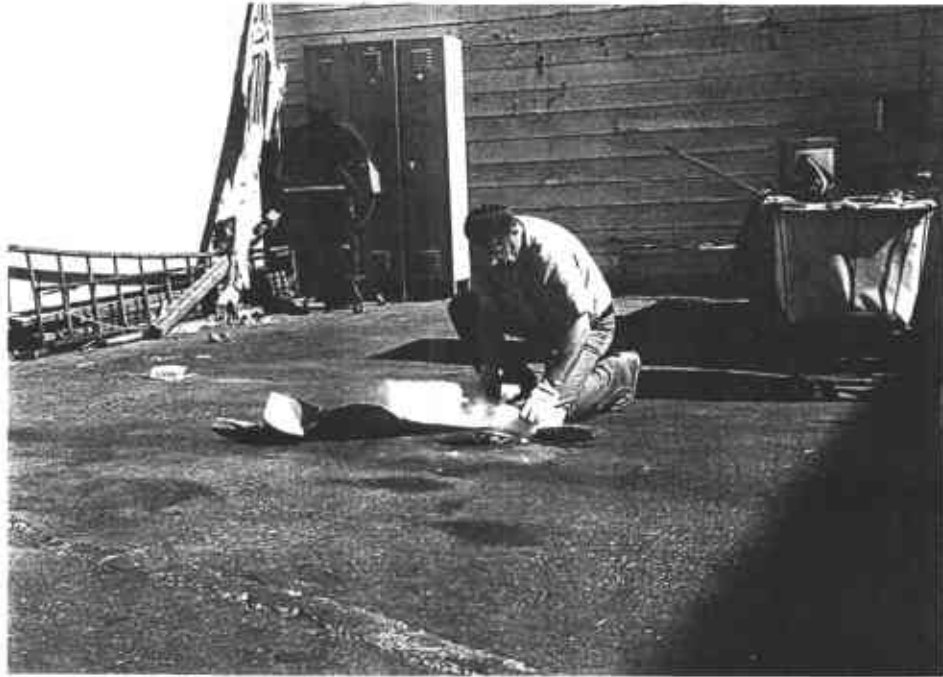
PHOTO 1: General view of UST Intake and preparation of dry ice Installation.
