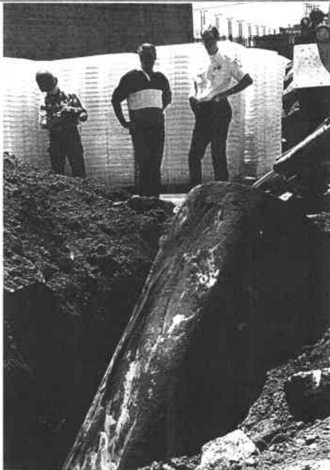
PHOTO 3: Upending of tank in excavation: Some breakage of tank occurred during removal.
