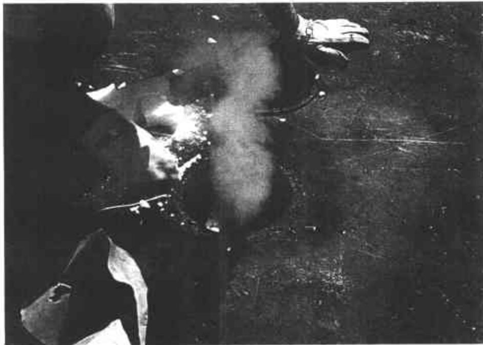
PHOTO 2: Dry Ice Installation into UST.
