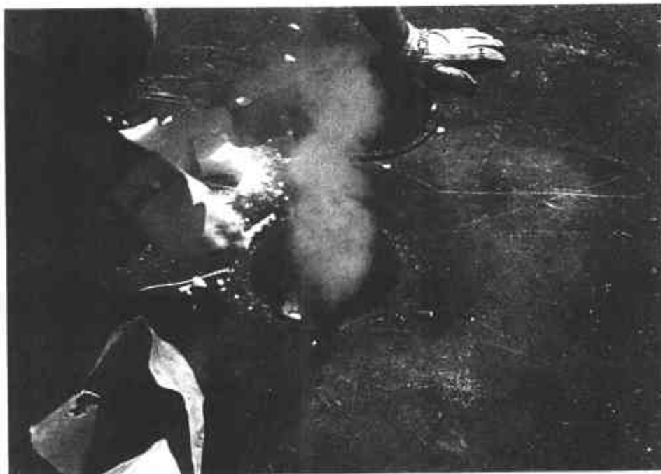
PHOTO 2: Dry Ice Installation Into UST.
