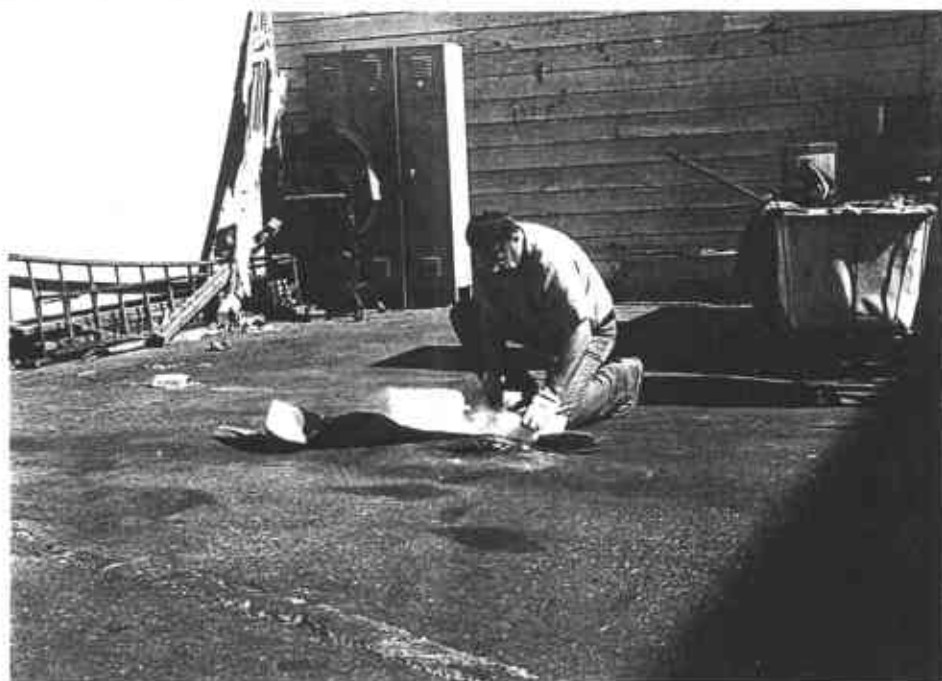
PHOTO 1: General view of UST Intake and preparation of dry Ice Installation.
