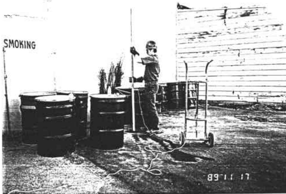
REDEVELOPMENT OF MONITORING WELL MW-2 WITH 2-INCH O.D. PVC BAILER
