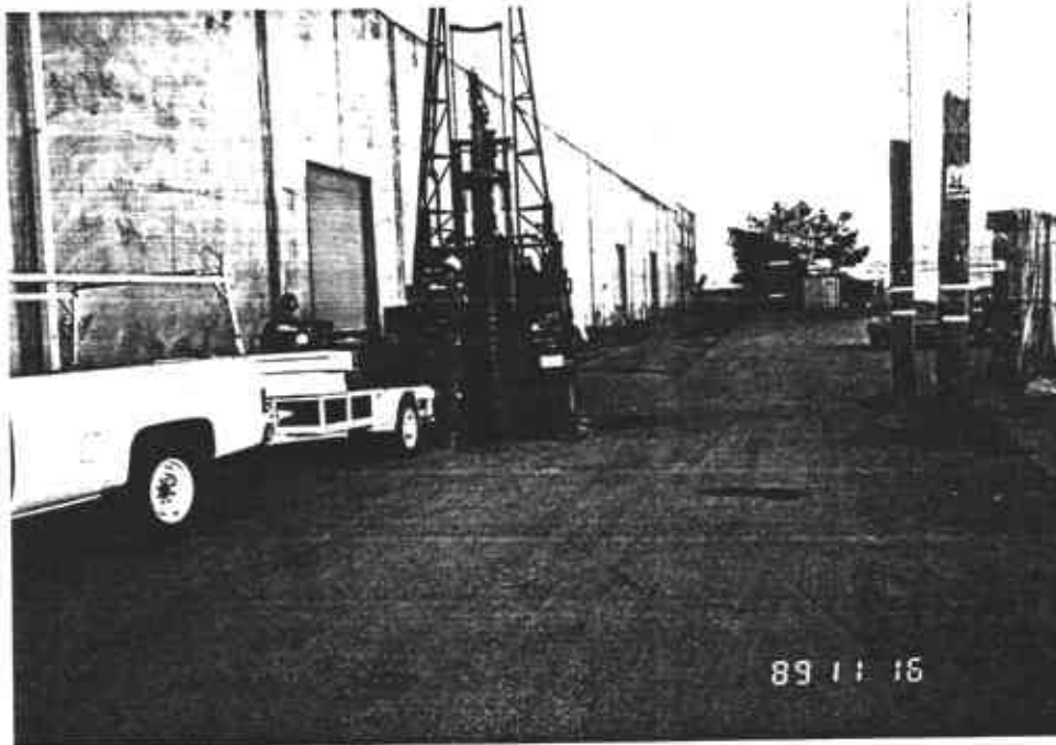
DRILLING PILOT HOLE FOR MONITORING WELL MW-5
