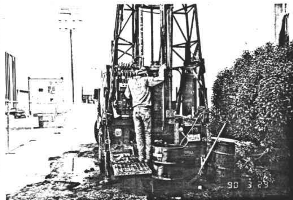
Well Development of Upgradient Monitoring Well MW-7.
