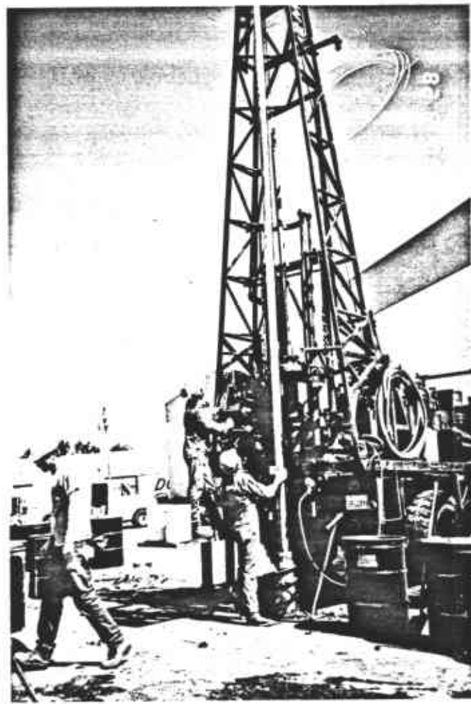
Installation of 4-inch ID Stainless Steel Well Casing and Screen, Extraction Well EW-1.
