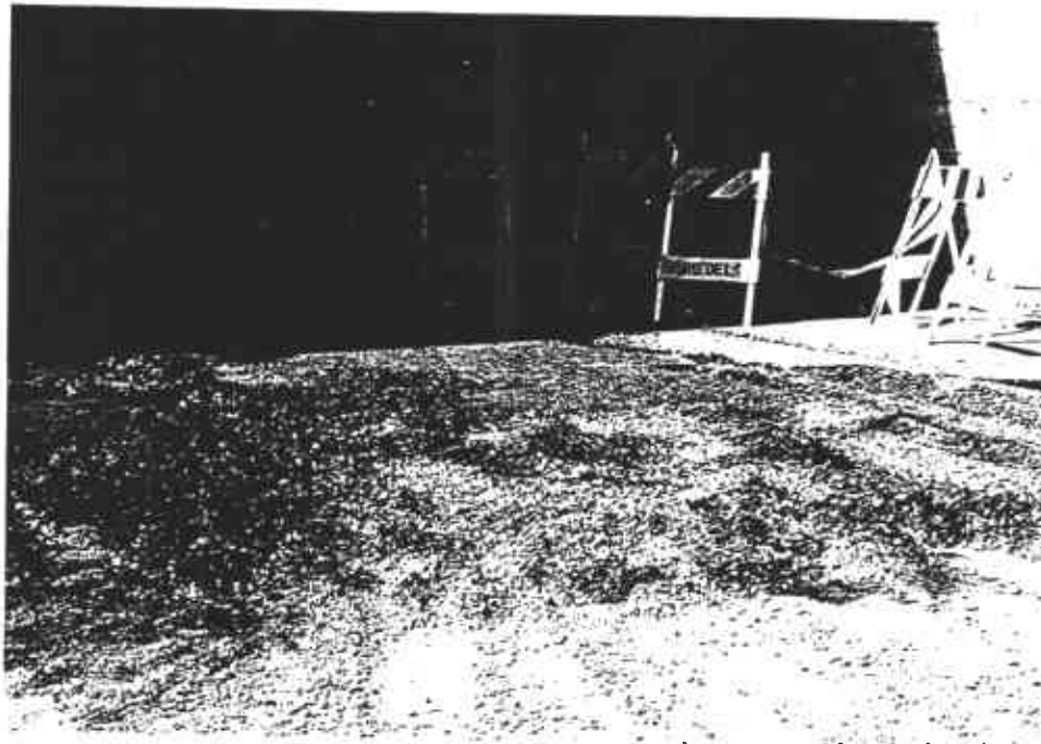
12. EXCAVATION BACKFILLING COMPLETED
