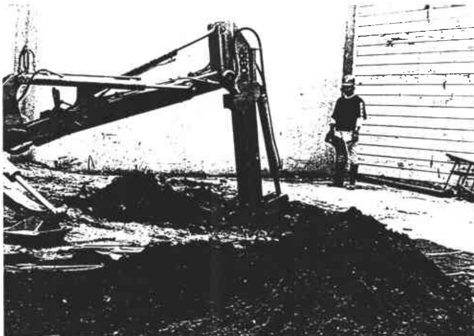
2. EQUIPMENT USED AND SITE EXCAVATION
