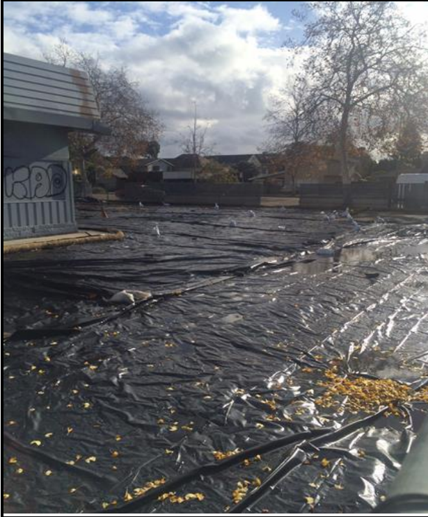
Plastic Covering Site After Excavation Completion
