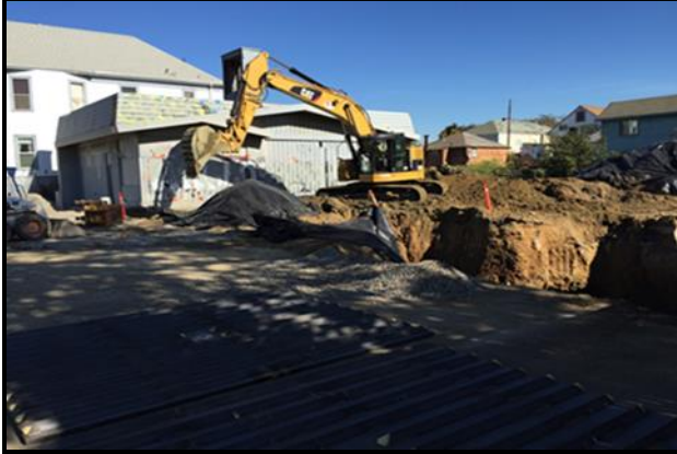
Excavator backfilling
