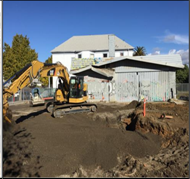
Backfilling near completion
