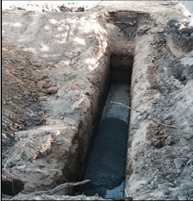
CDF Slurry Wall at Southern Boundary
