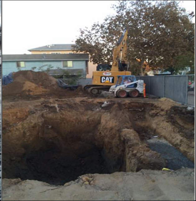
Open excavation with CDF Slurry Wall
