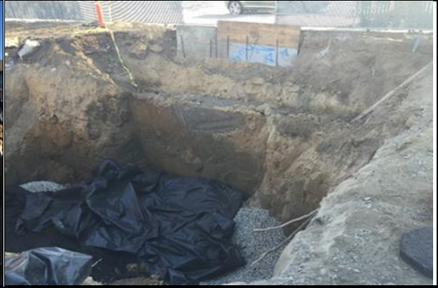
Excavation partially backfilled
