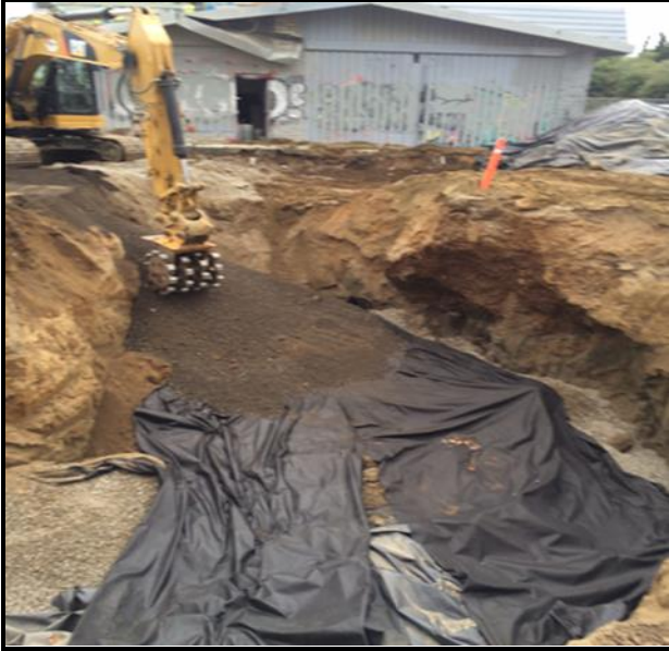
Compaction of backfill with Sheep's Foot Roller
