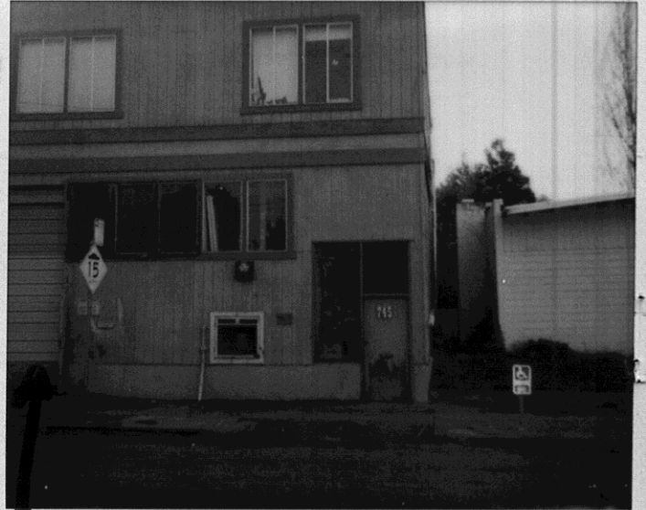
← 20' → MWT located ~ 20' from rhd of bldg.
