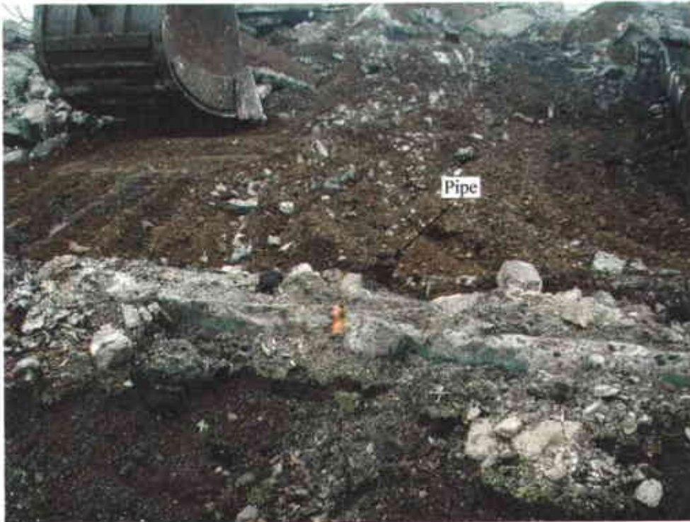
Photograph 1: Foundation of Building 303, showing pipe (looking west).
