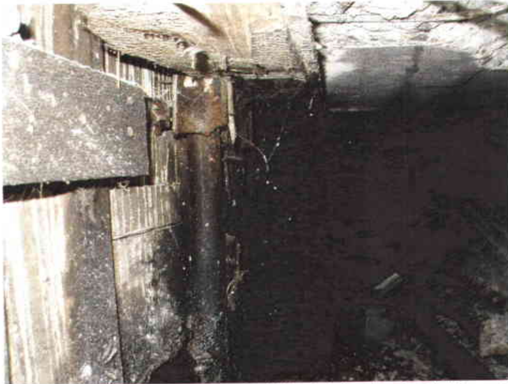
Photograph 3: Corner of foundation of Building 301 showing pipe (looking south).
