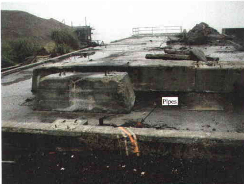
Photograph 2: Pipes underneath foundation of Building 303 (looking west).
