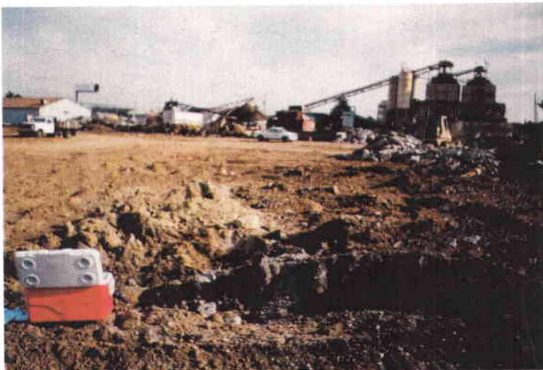
Photograph 6: Former tank location (looking south).
