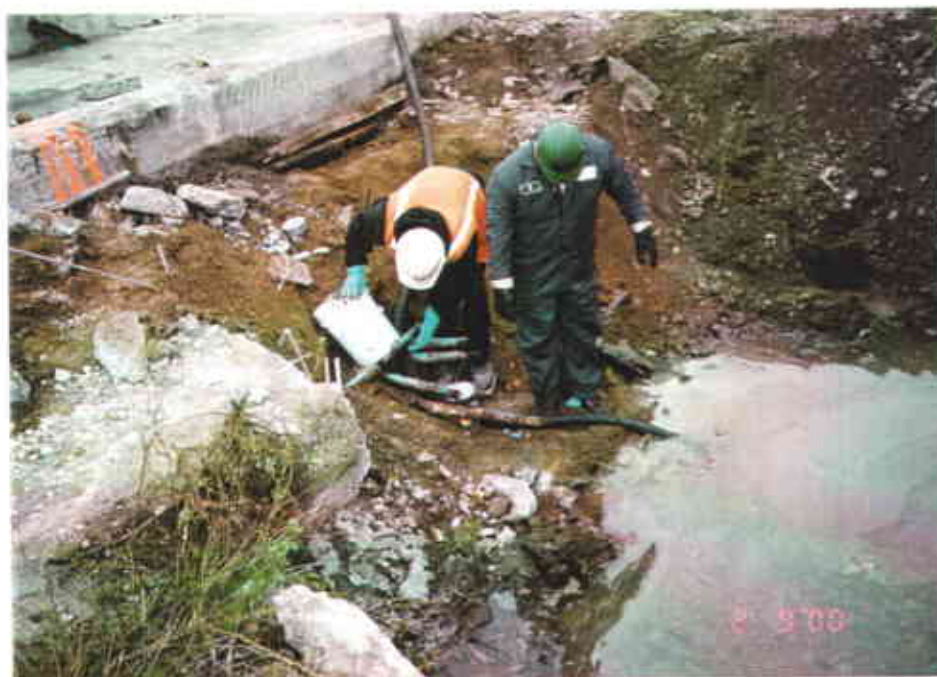
5B: Sealing pipeline ends and vacuuming excavation.
