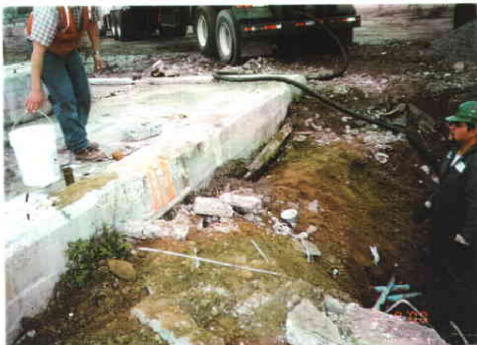
5A: Flushing pipelines.
