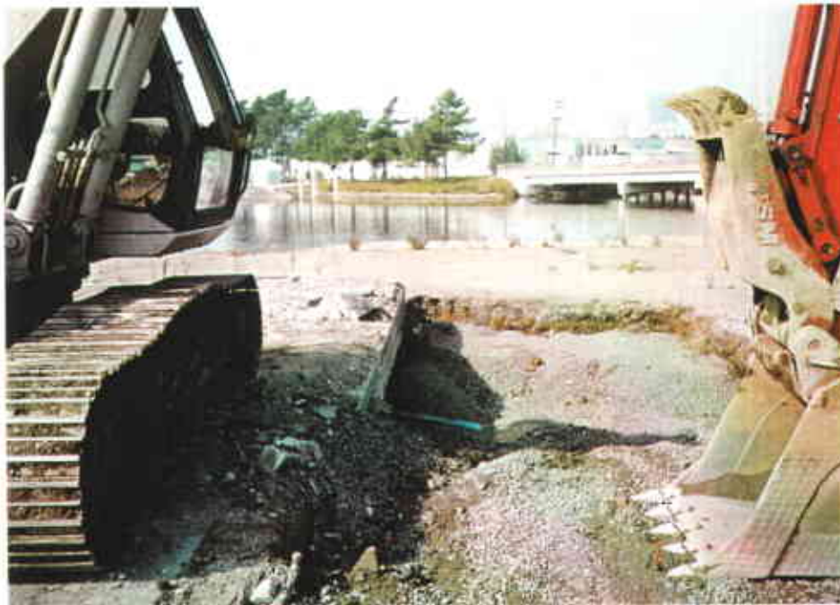
8B: Backfilling the excavation.
