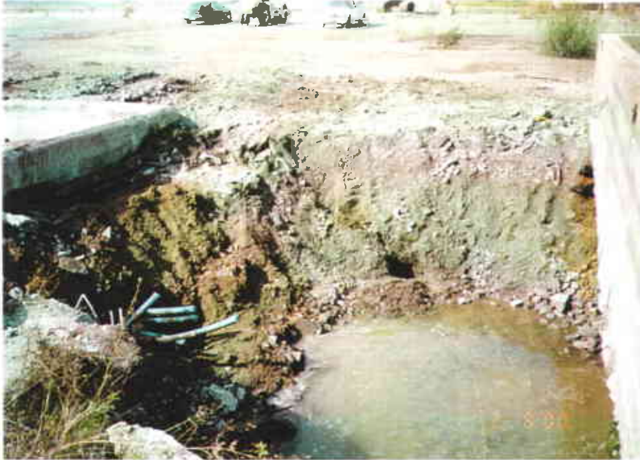
4A: Excavation and pipes.
