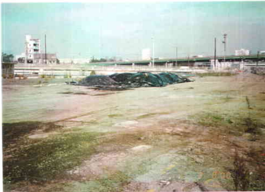
4B: Excavated backfill stockpiles.
