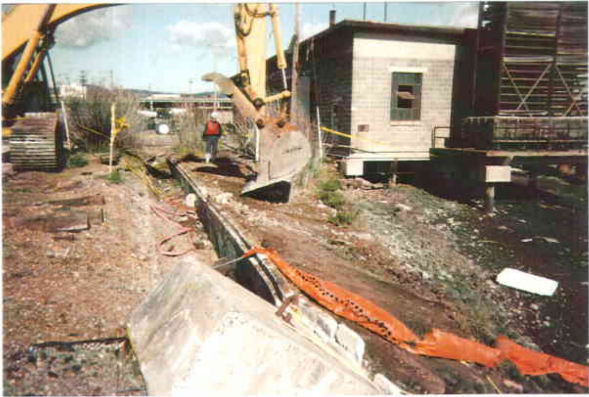
11. Sandblast grit and debris removal activities in the southeast supra-tidal zone.
