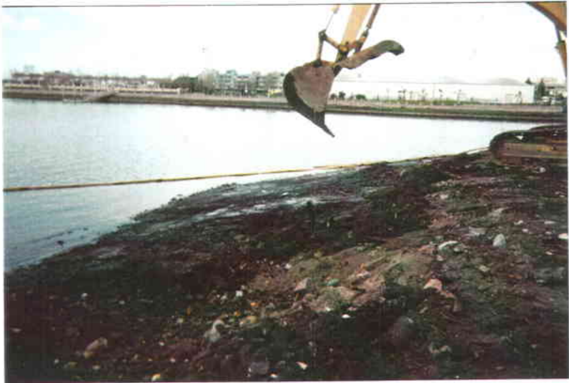
9. Sandblast grit and debris removal activities in the southwest supra-tidal zone.
