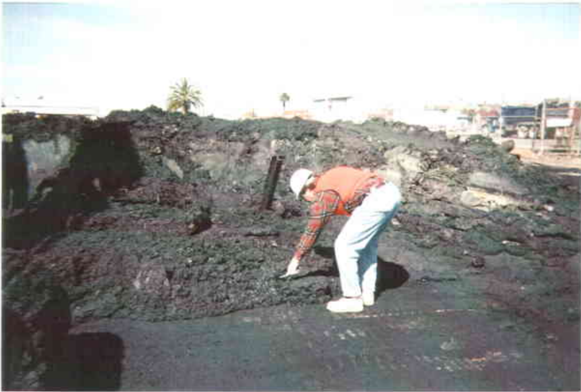
9. Air emissions monitoring of the stockpile during trans-loading activities.
