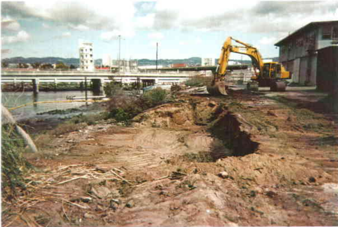
5. Photograph showing northwest supra-tidal zone sandblast grit and debris removal area.
