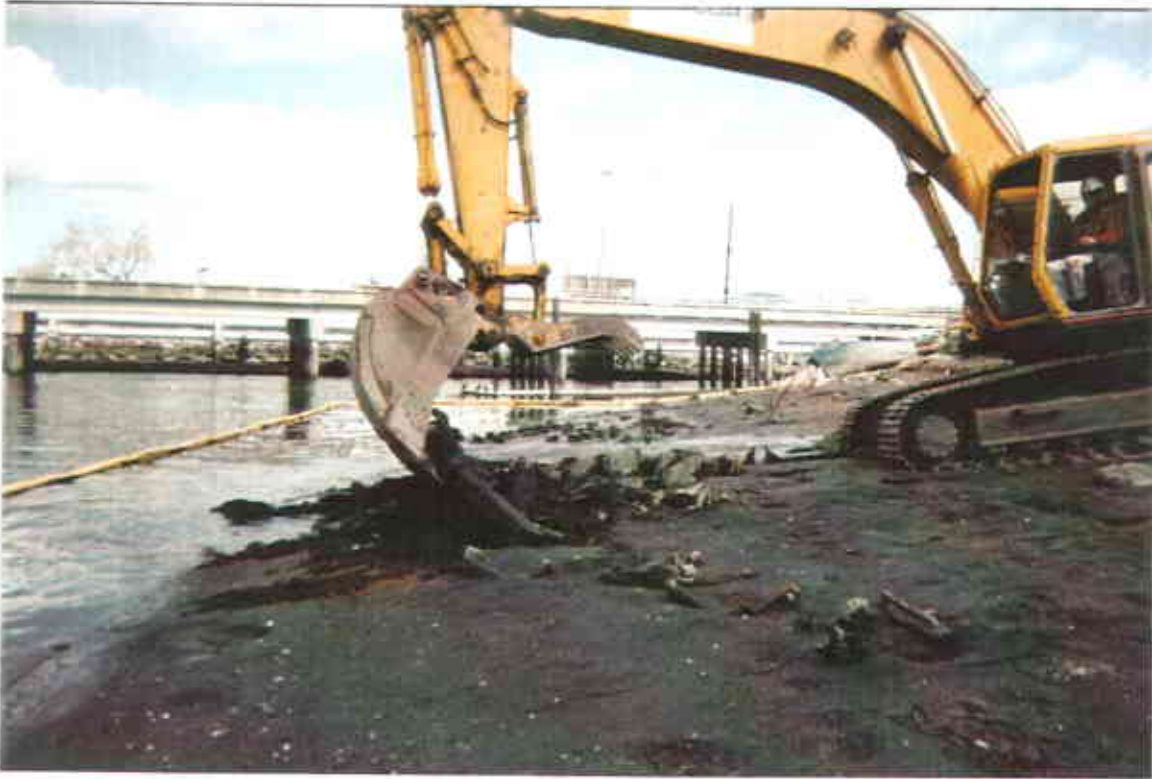
1. Sandblast grit and debris being removed from the northwest inter-tidal zone.
