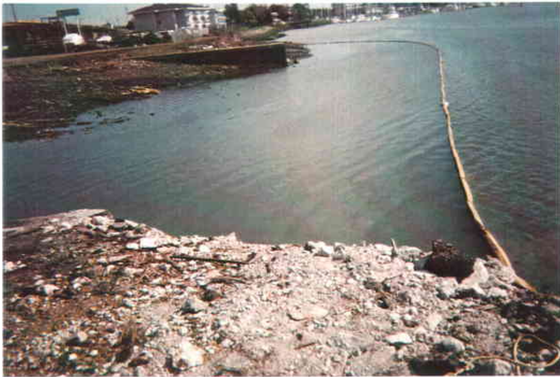
12. Photograph of containment boom in place during removal activities.
