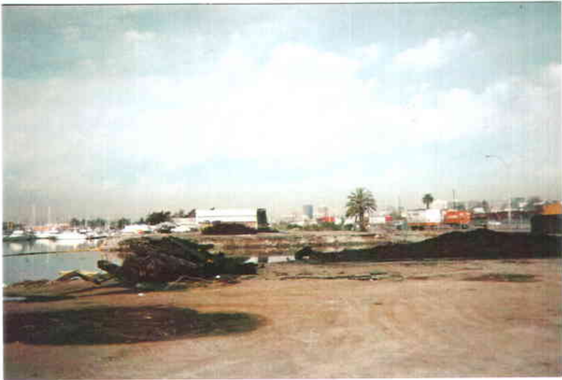
11. Photograph showing debris and sandblast grit stockpiles in foreground, trans-loading activities in background
