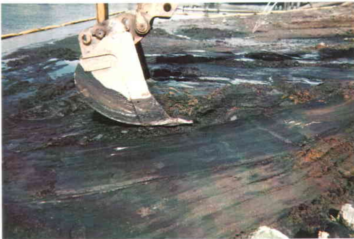
2. Photograph showing sandblast grit being removed from the northwest inter-tidal zone, exposing the bay mud.
