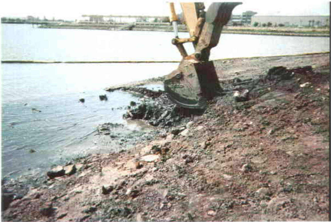
7. Sandblast grit and debris removal activities in the southwest inter-tidal zone.
