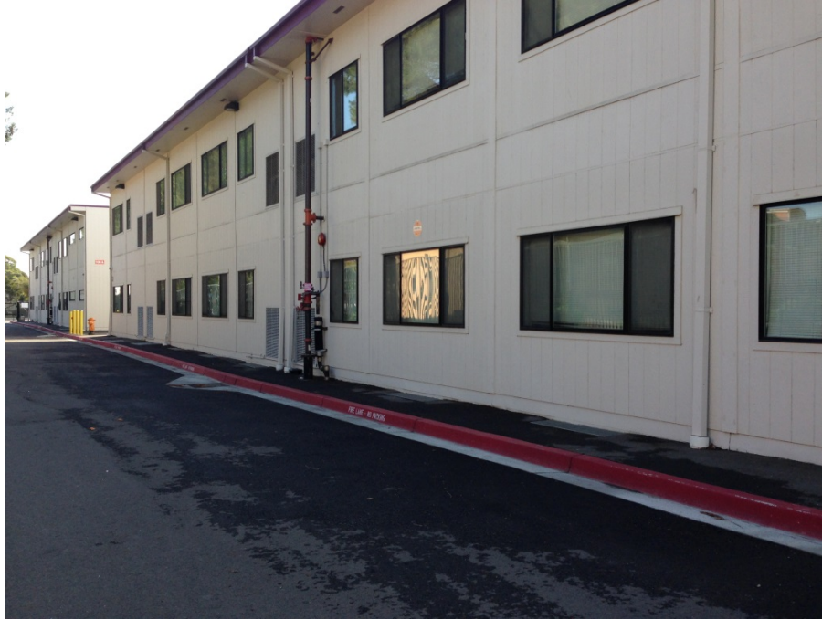
Photo 1 – Building 200 facing south, adjacent to the road.
