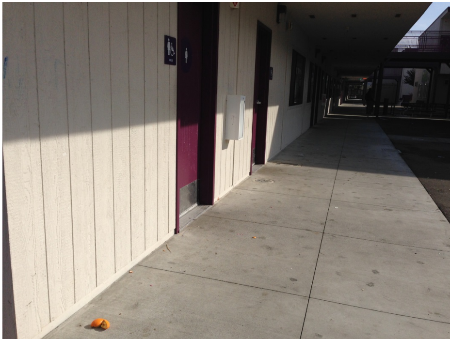
Photo 2 – Building 200 facing north – no crawl space air vents
