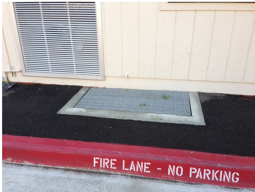
Photo 4 – 4 feet (length) by 2 feet (width) access/vent well crawlspace
