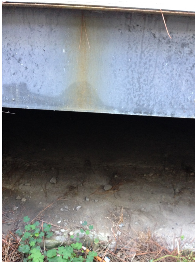
Photo 5 – Crawl space below grade, underneath the metal grille
