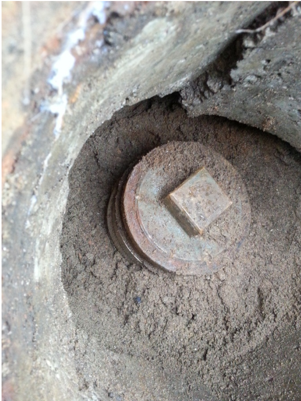
View inside sewer cleanout/vault
