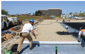
2. Geo-Seal BASE is a composite sheet material comprised of HDPE and non-woven geotextile
