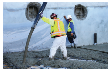
6. Concrete is placed directly onto the completed Geo-Seal system
