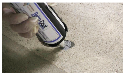
2. Retro-Coat Gel and fillers are used to repair concrete cracks and other imperfections
