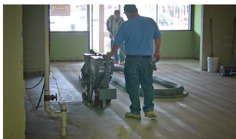
1. Existing concrete slab is first cleaned and then abraded
