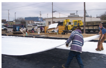
5. Geo-Seal BOND is applied over the Geo-Seal CORE to provide additional protection
