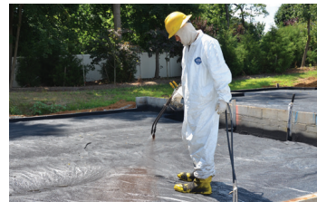
3. Geo-Seal CORE is spray applied to increase the systems tensile strength and provide a seamless membrane
