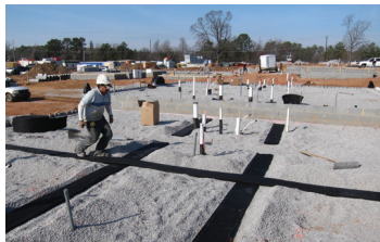
1. Vapor-Vent should be installed in a permeable subgrade to maximize vapor collection ability
