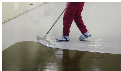
4. Retro-Coat is applied to a nominal thickness of 20 dry mils
