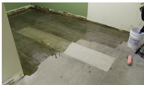
3. Retro-Coat PRIMER is applied to the concrete surface as final preparation. This increases adhesion between the concrete slab and the Retro-Coat, as well as address moisture vapor transmission.
