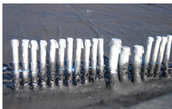
4. Penetrations are sealed individually
