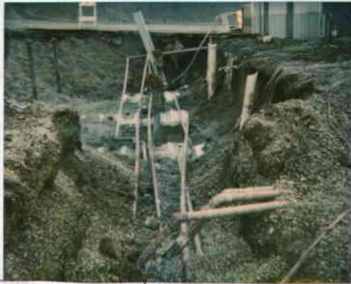
3530 MacArthur 4/26/94 Gas product piping to existing gas USts Rinsed 09318221467-2 0547 1736 Subject Site
