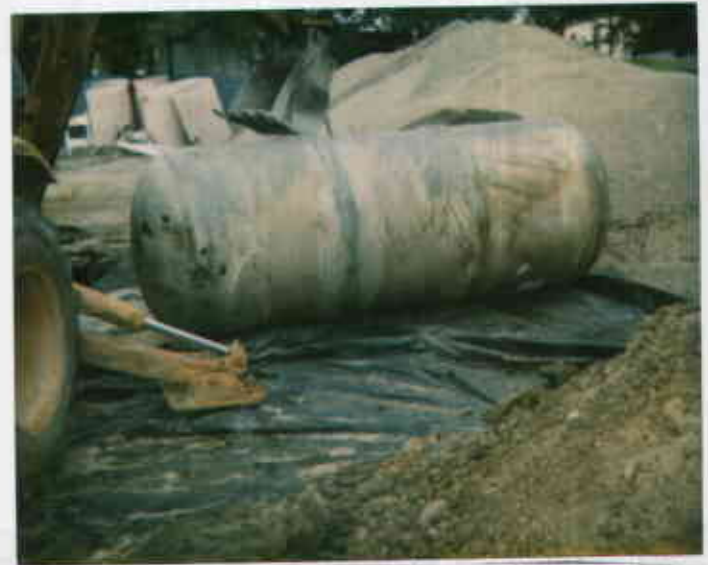
3530 MacArthur, Oakland 5/19/94 1,000-gallon fiberglass waste oil UST removed. 85318221467-2 No apparent holes. 85318221467-2 Juliet Shur
