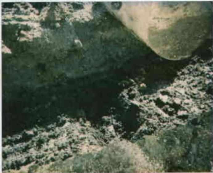
3530 MacArthur, Oakland 5/2/94 Sample location PX-1 from overexcavated trench 09318221467-2 0547 1732 Juliet Shinn
