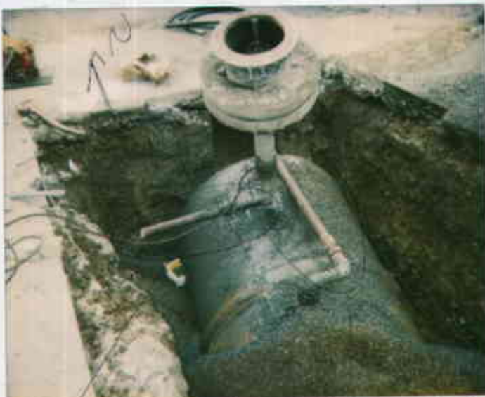
3530 MacArthur, Oakland 5/19/94 1,000-gallon waste oil UST. Vent line gone north. 85318221467-2 Remote fill going east/west. 85318221467-2 Juliet Shur
