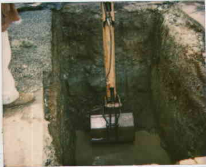
3530 MacArthur, Oakland 5/19/74 12215117976-B South wall of waste oil pit where one sample collected (at ~6' deep) Juliet Shen
