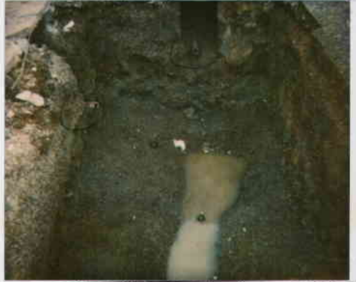
3530 MacArthur, Oakland 5/19/94 12215117976-8 Groundwater in waste oil UST pit Stained soil on sidewalls at ~6' deep. Juliet Shur
