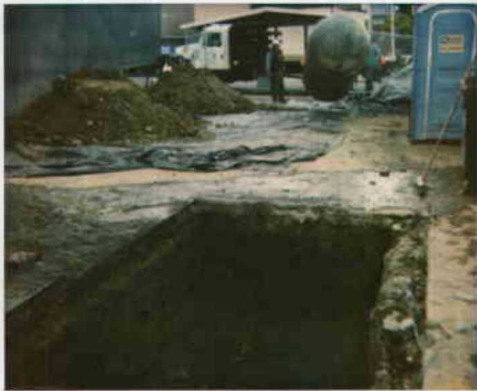
3530 MacArthur, Oak 12215117976-8 5/19/94 Waste oil UST pit w/ stockpiled soil in background. Tank hauled by Erickson Juliet Shur
