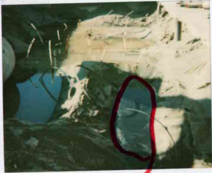
no product on surface of water, where former w.o. UST was.
