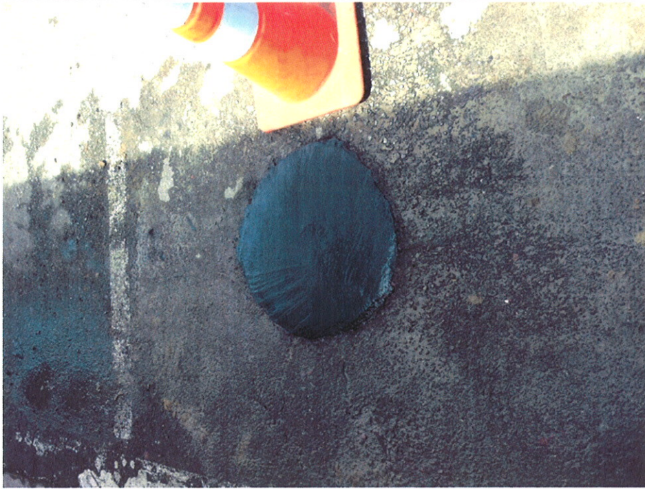
View of MW-3 after destruction and seal.
