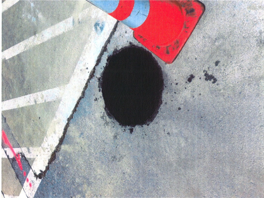
View of MW-1 after destruction and seal.
