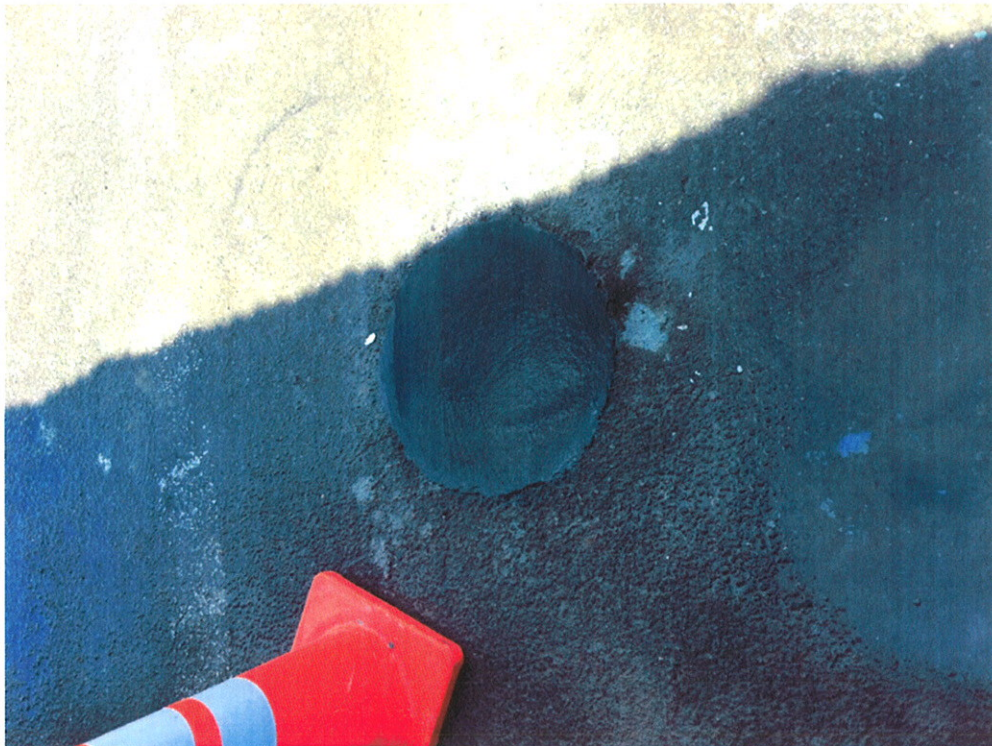
View of MW-4 after destruction and seal.
