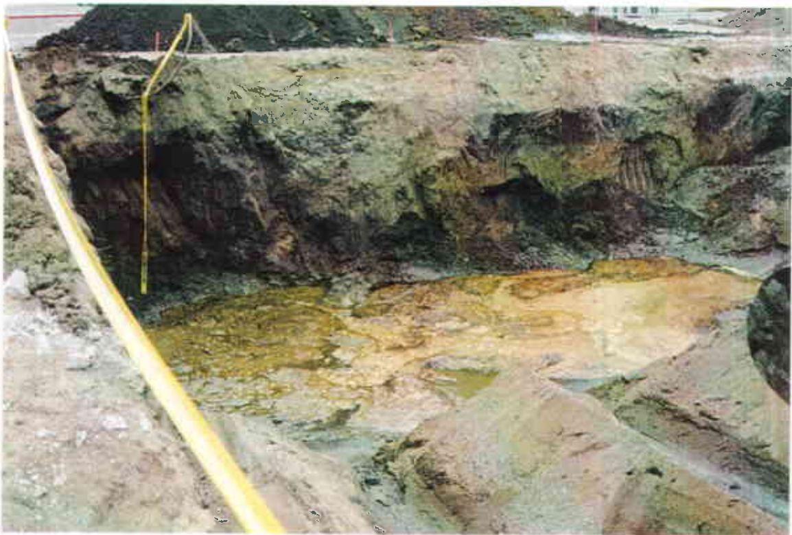
D) View of the tank cavity overexcavation.
