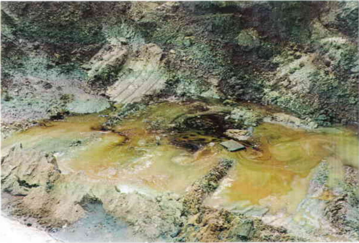
E) View of tank cavity overexcavation and floating product.
