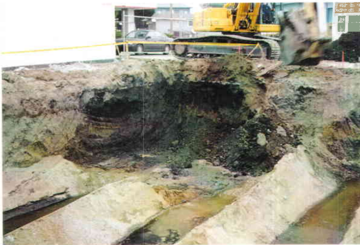
B) View of the tank cavity and floating product, orientated to the northeast.
