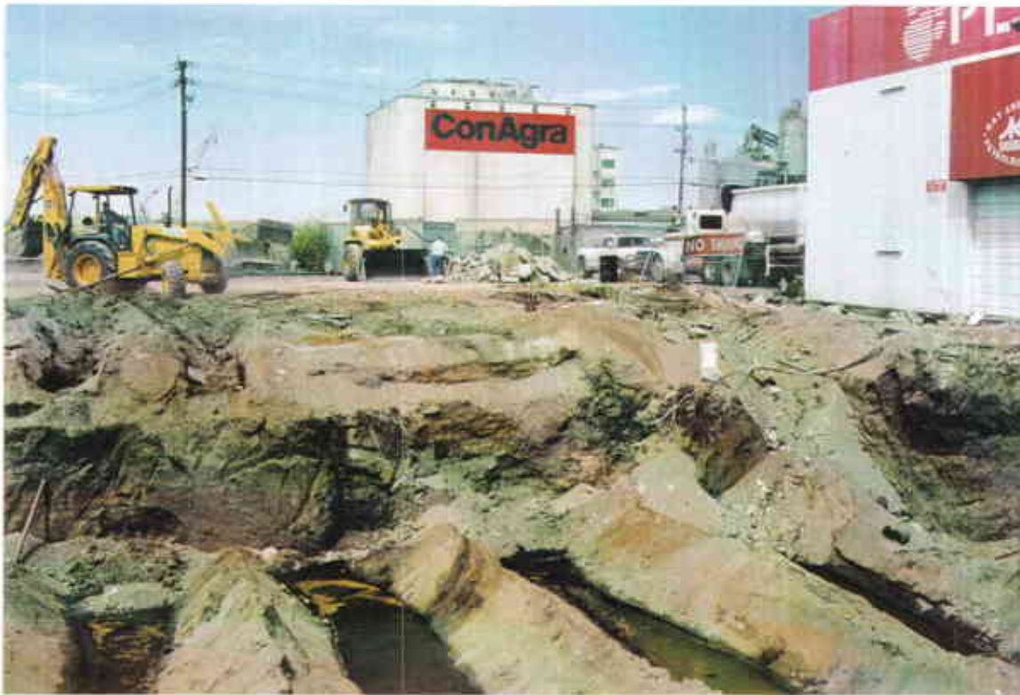
A) View of the tank cavity orientated to the west.
