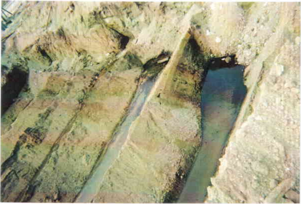
C) View of the tank cavity and floating product (Tank 1 was in the foreground).
