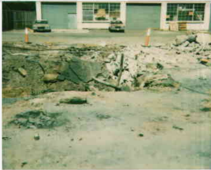
former dispenser island 501 5th St Oakland, 9/14/92
