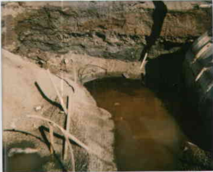
333 @ 8 th Brown slurry on PCC 11/4/93 Surface of G.W.
