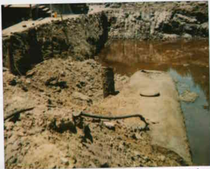
054163023672W 7/10/95 505MAA 0539 8960 Exposed The diesel tank being vacuumed out
