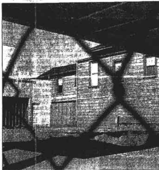
The former Bill Chun service station at the corner of... been vacant for three years.
