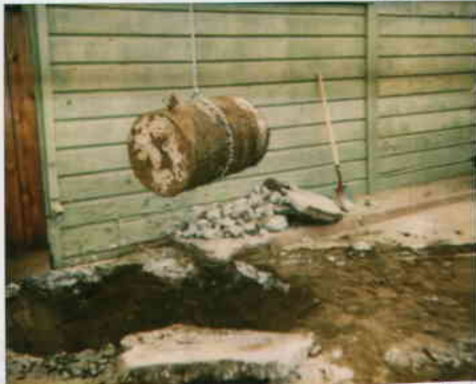
2301 Santa Clara Ave, Alameda 11/16/95 05517303103-24 2785 0211 COPIES & ENLARGEMENTS CALL 800-421-1030 55-gallon drum converted into waste oil storage - Juliet S.
