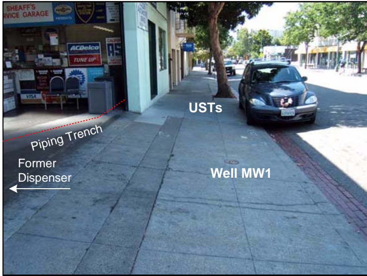
Photograph No. 4 – View of College Avenue to right & subject property (green building with large rollup door). USTs formerly located in sidewalk near tree. Monitoring well MW1 in driveway/sidewalk. Former product piping trench to former dispenser inside of rollup door to left.
