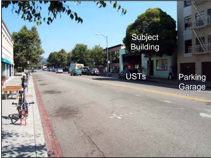
Photograph No. 1 - Street scene looking northward uphill on College Avenue showing subject building (green building with large rollup door & tree) on right. Newer commercial development across street on left. Storm drain - 96" diameter - flows down middle of street with uphill to left. USTs formerly located in sidewalk under tree.
