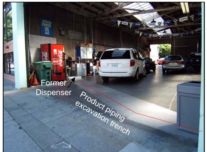
Photograph No. 8 - Interior view of subject building at 5930 College Avenue with rear storage yard beyond open doorway at rear of photograph. Concrete patch of product line excavation in foreground with former dispenser location at concrete pad on left wall of building.
