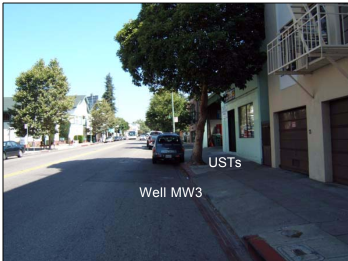
Photograph No. 3 - View northward of College Avenue and subject property to right behind tree. Adjacent property at 5920 College Ave. to right with first floor parking-retail (T-Mobile store) and multi-family above. USTs in sidewalk under tree and monitoring well MW3 in street.
