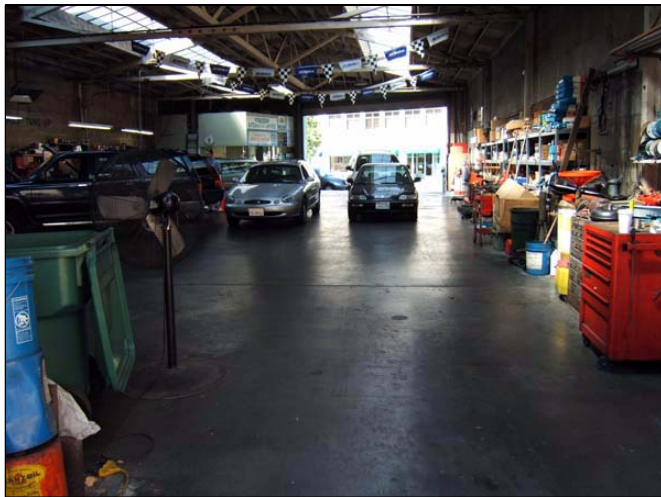
Photograph No. 6 - Interior view of subject building at 5930 College Avenue occupied by Stauder Automotive Service. College Avenue beyond rollup doorway. View from doorway to rear storage yard.
