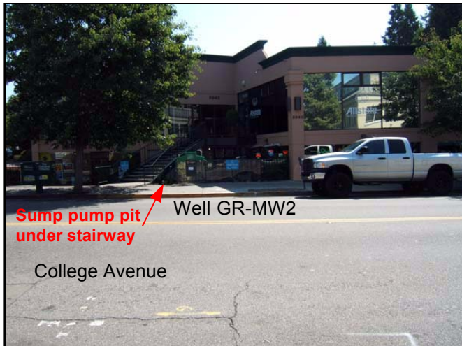
Photograph No. 9 - View of adjacent commercial building at 5940 College Avenue occupied by Barclays Restaurant & Pub and commercial businesses. Former Chevron service station. Development is 3 feet below grade with sump pump pit located at left of picture beneath stairway. Gettler-Ryan well GR-MW1 in sidewalk near sump pump pit.
