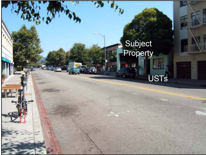
Photograph No. 1 - Street scene looking northward up College Avenue - subject (green building with large rollup door) and adjacent buildings on right. Newer commercial development across street on left. Storm drain - 96" diameter - flows down middle of street with uphill to left. USTs formerly located in sidewalk under tree.
