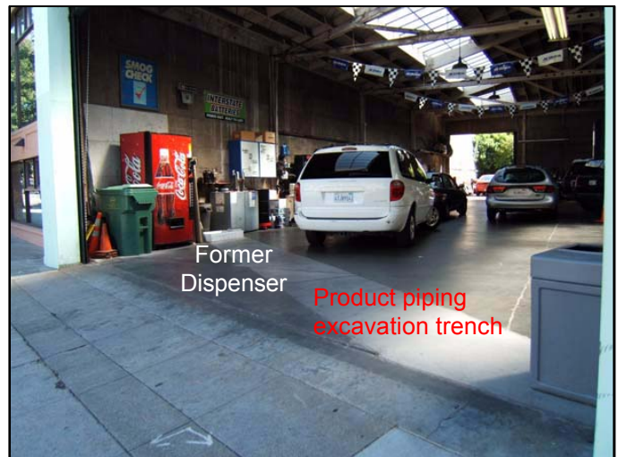
Photograph No. 8 - Interior view of subject building at 5930 College Avenue with rear storage yard beyond open doorway at rear of photograph. Concrete patch of product line excavation in foreground with former dispenser location at left of photograph.
