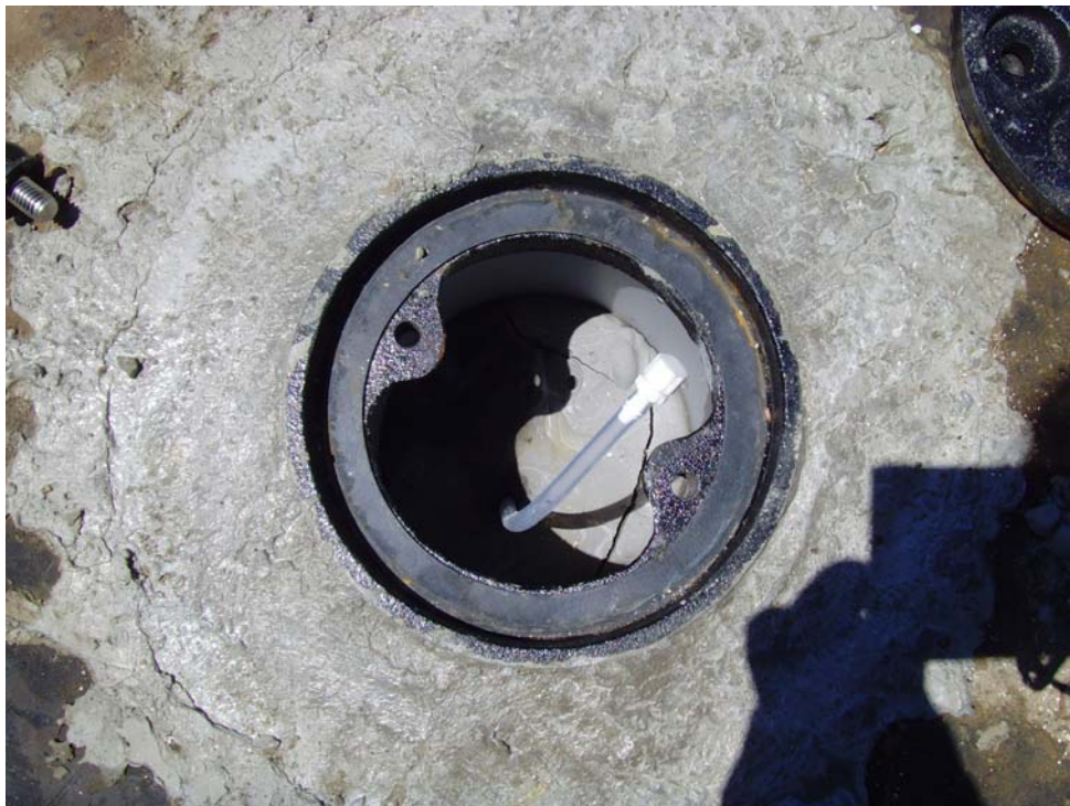
View of soil gas probe installation
