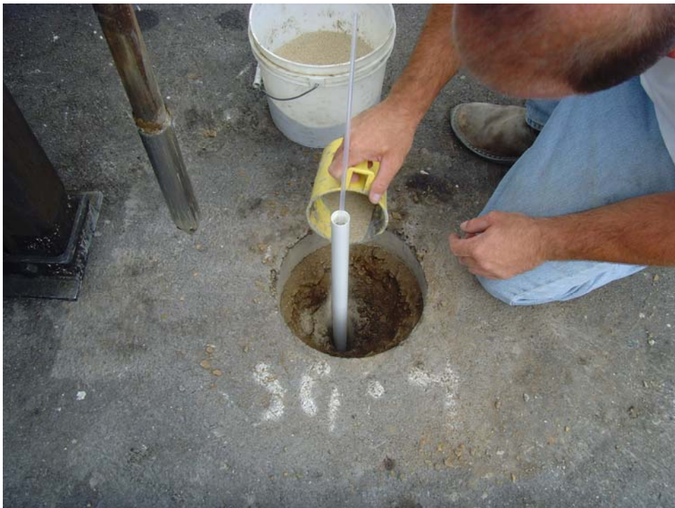
View of placement of sand pack around polytube
