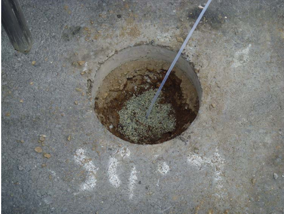
View of soil gas probe installation
