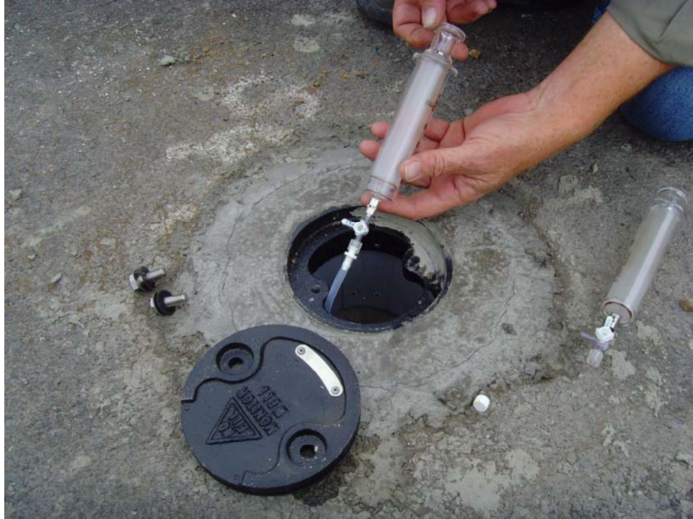
View of soil gas probe sampling
