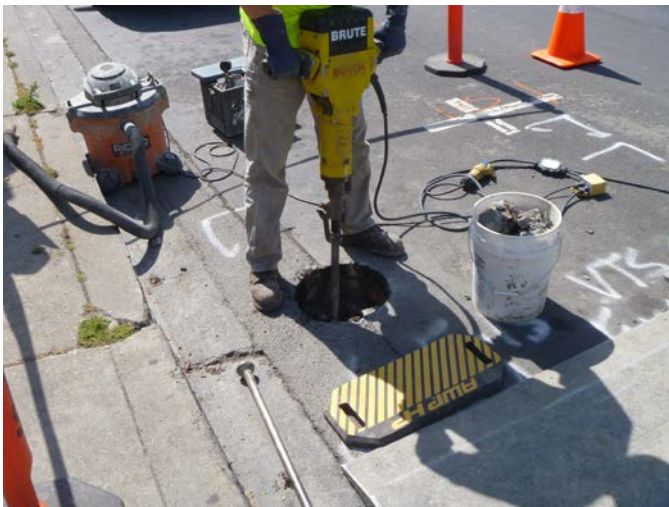
Removing well boxes and associated concrete
