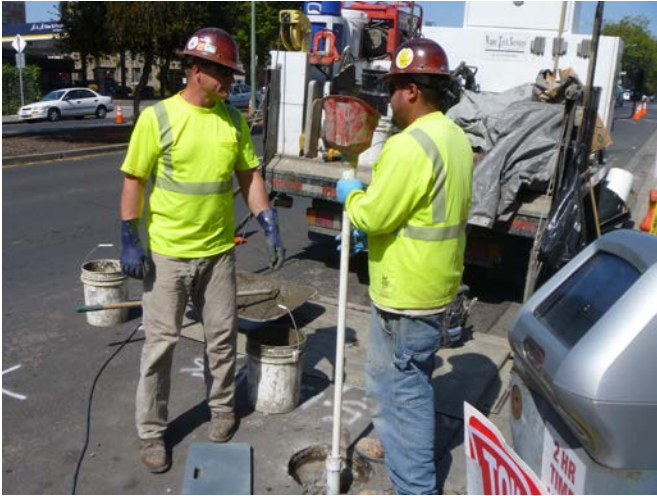
Removing well boxes and associated concrete
