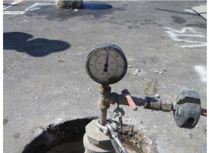
Pressurizing and maintaining above 25 PSI for a duration of five minutes
