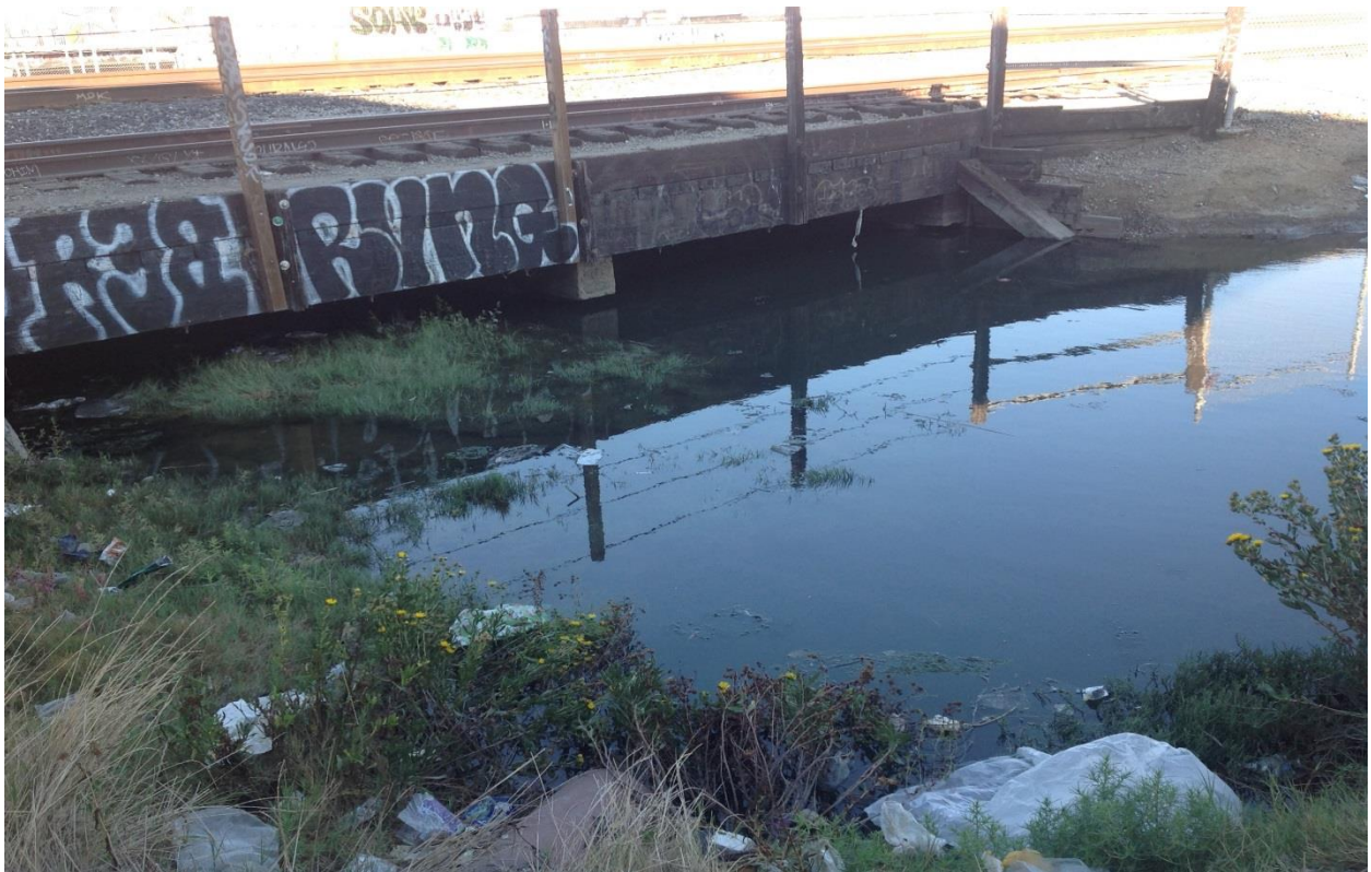
Photo 2: Eastern water quality survey spot (looking east) at evening high tide.
