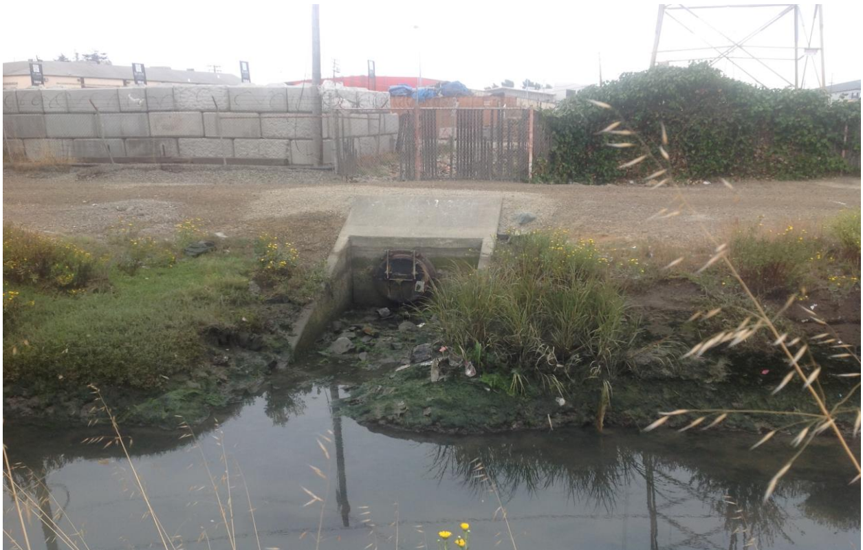
Photo 8: Storm water drain outlet within Seminary Creek coming from drainage canal south of the creek along the western edge of the site.
