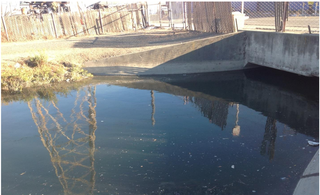
Photo 4: Western water quality survey spot at evening high tide.
