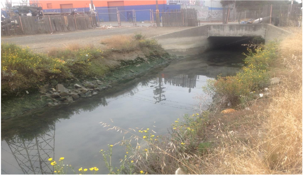
Photo 3: Western water quality survey area (looking west) at mid-day low tide.
